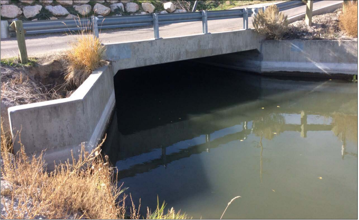
T-2 Upstream View (C-1 North Jordan Canal)
