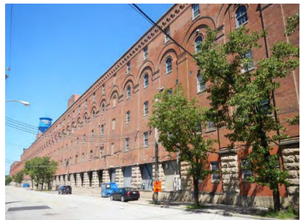
B&O Freight Terminal/Longworth Hall, looking west along Pete Rose Way.
