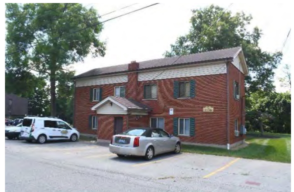
Colonial Revival-inspired four-plex apartment building in the proposed Elberta Apartments Historic District.
