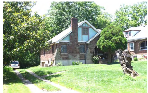
Tudor Revival house at 53 Rivard Drive that is a contributing resource to the proposed Hillsdale Subdivision Historic District.
