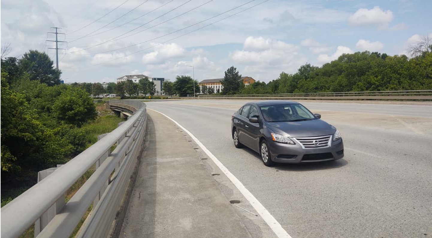
Hector Henry Greenway Bridge Crossing at Rocky River
