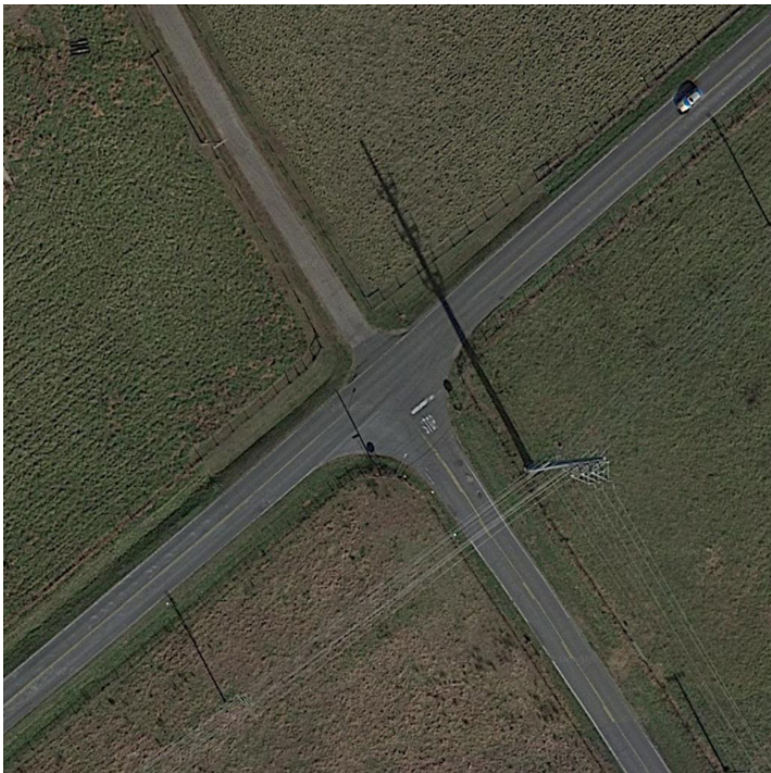
Concord Farms Road Existing Conditions
