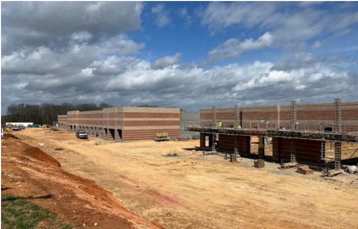
Springs Business Park - Under Construction
