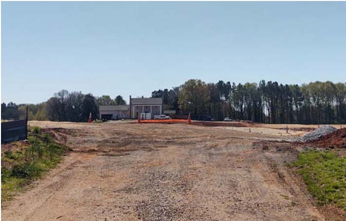
Olde Homestead Construction - Under Construction
