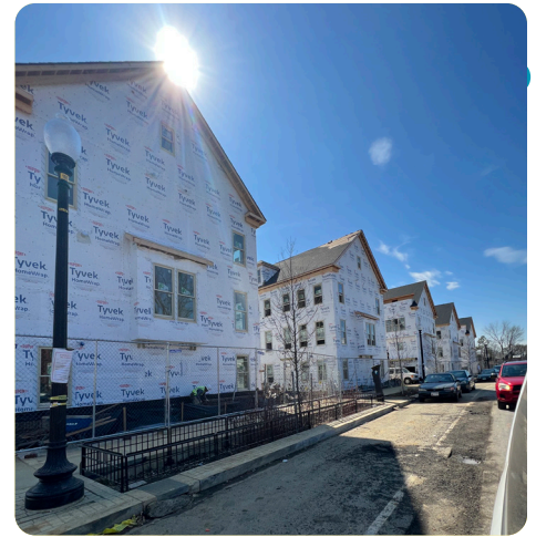
Townhouses under construction at St. Elizabeths
