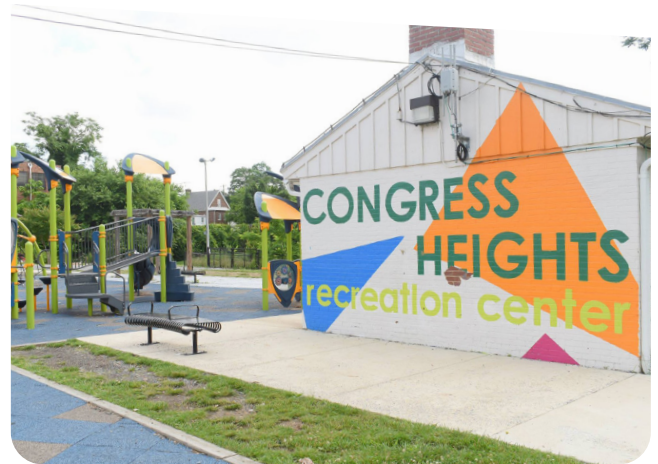
Existing Congress Heights Recreation Center
