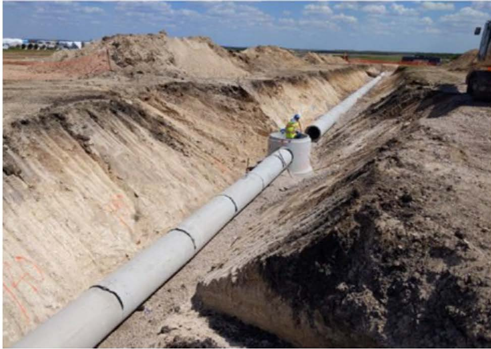
Stormwater system installation
