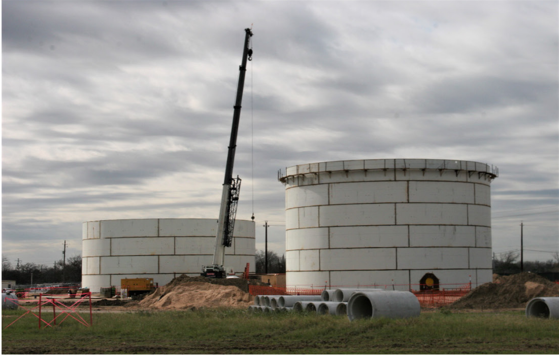
Storage tanks walls under construction.
