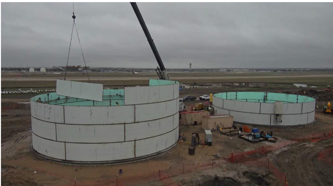
Tank steel wall construction has begun.
