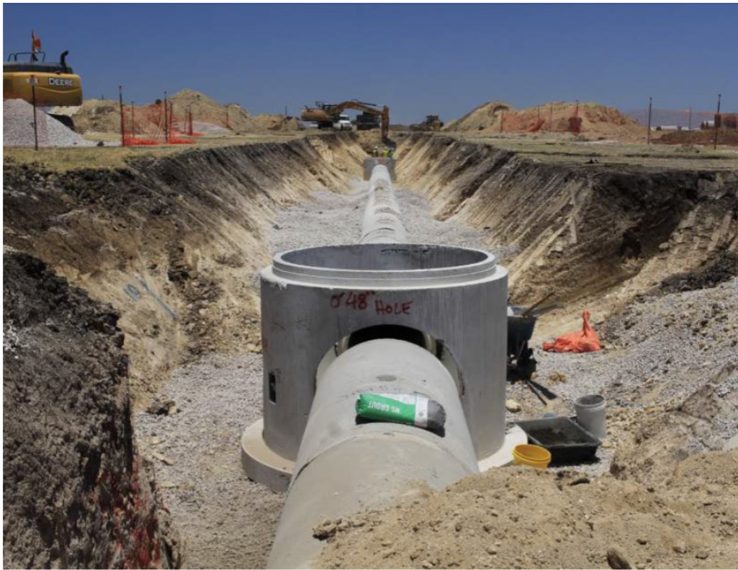
Stormwater system installation
