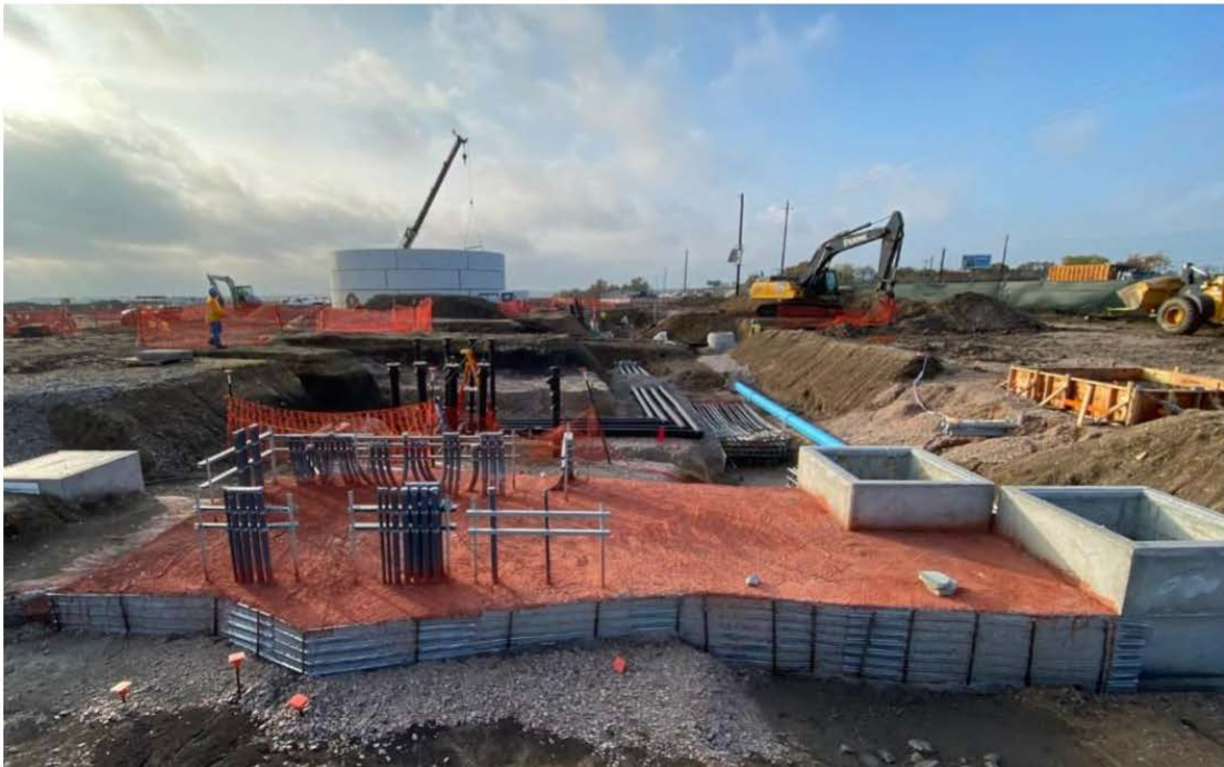
Fire foam building subgrade being prepped.
