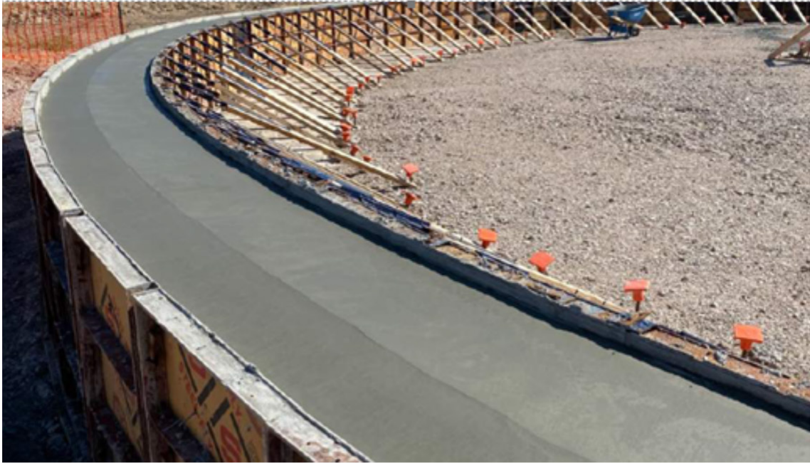
Tank #101's concrete foundation
