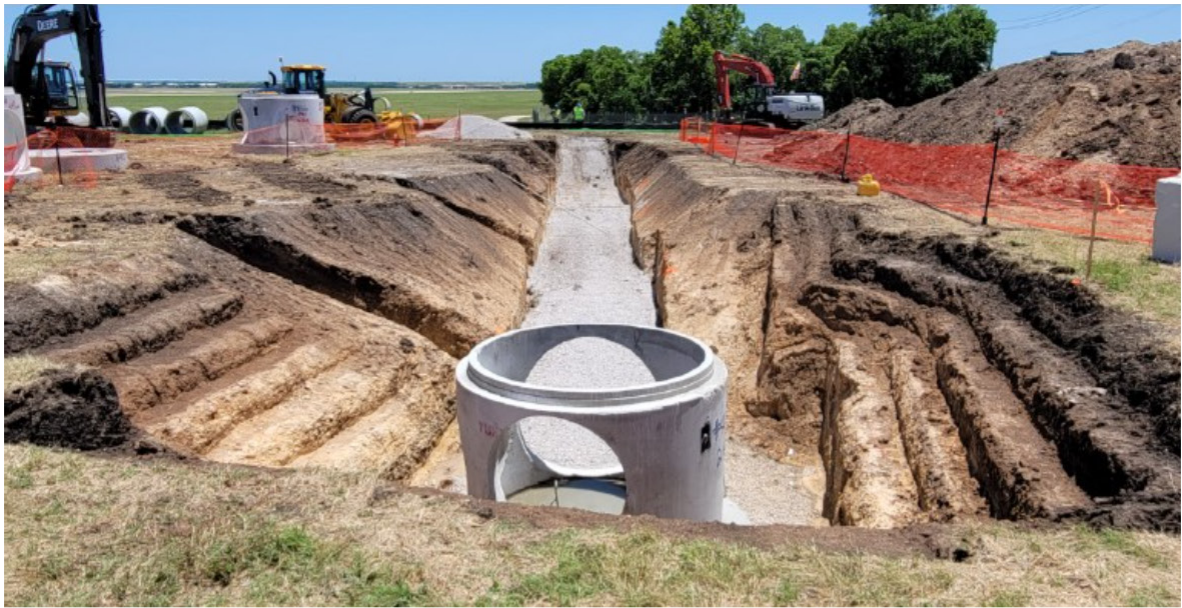
Stormwater manhole installation
