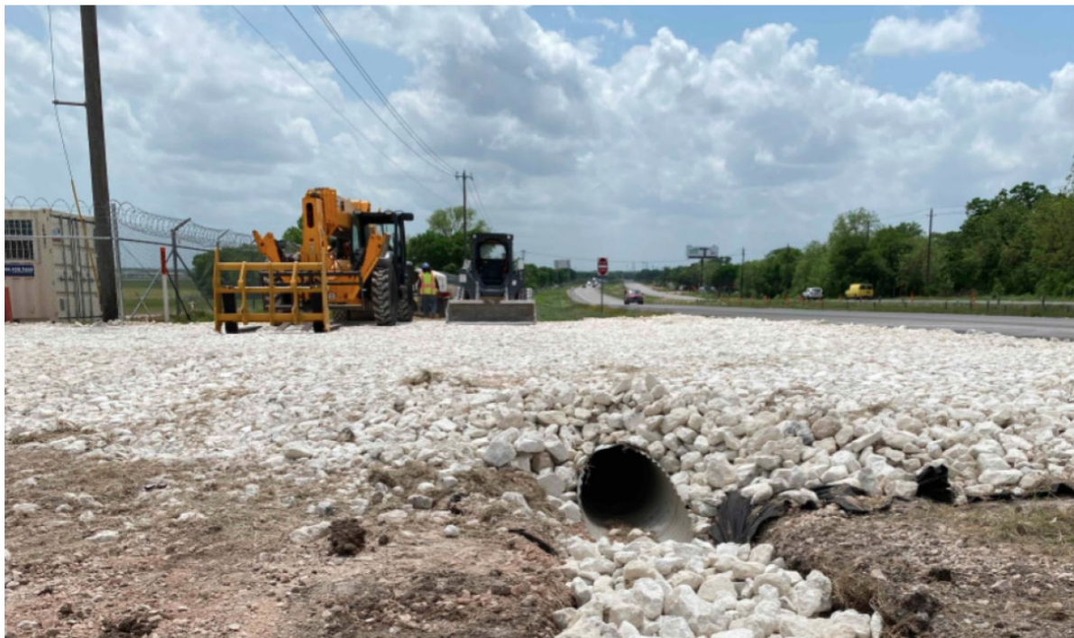
Temporary construction entrance
