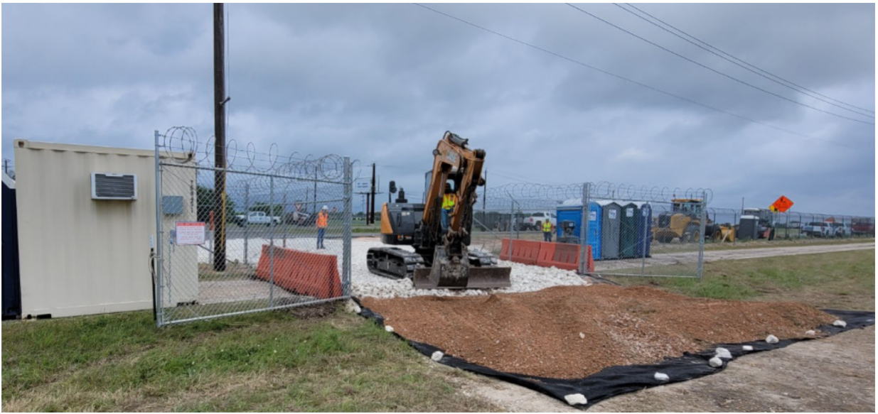
Temporary construction entrance
