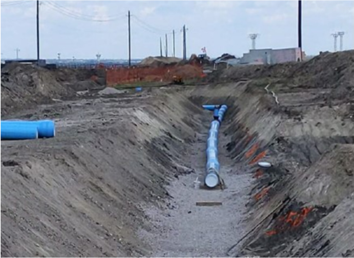
Water line installation.
