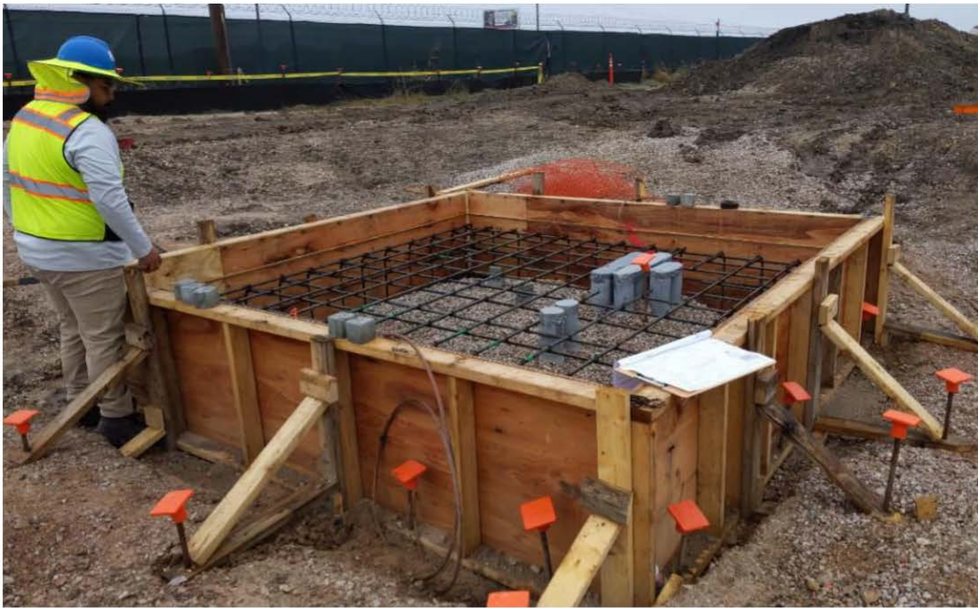
Building transformer pad work
