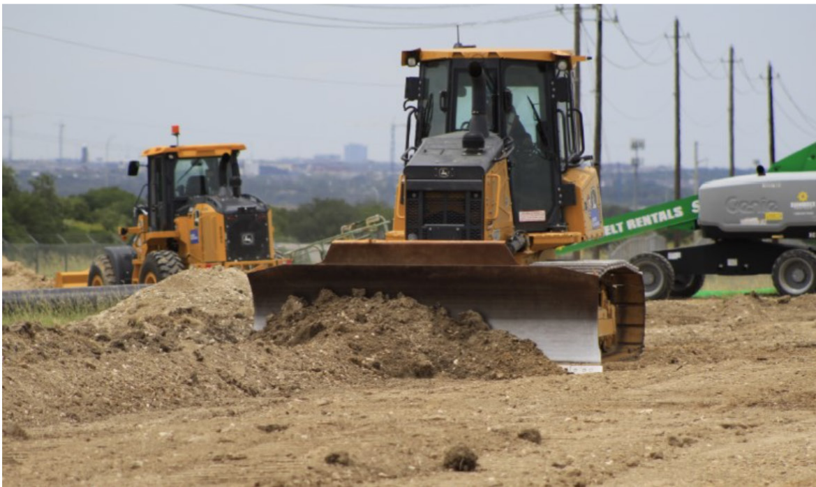
Grading for new airport perimeter road
