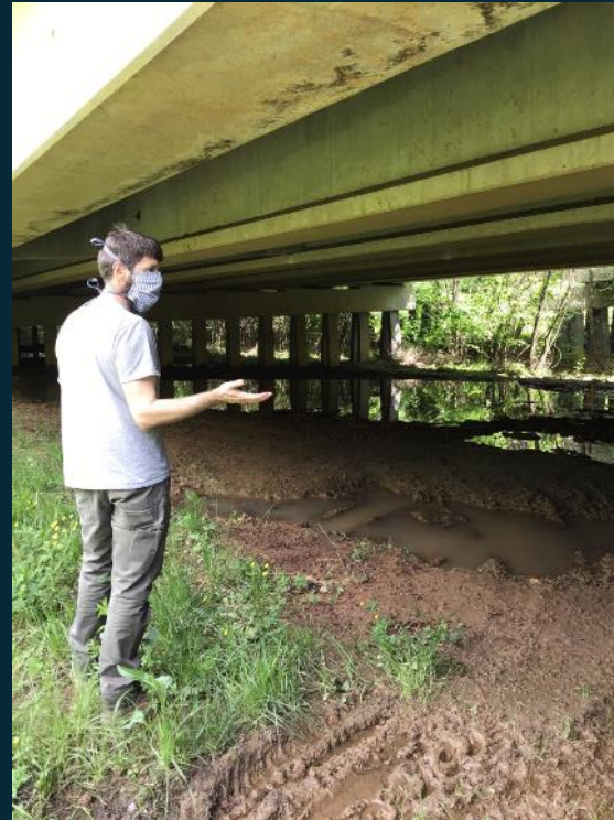
Western I-485 underpass
