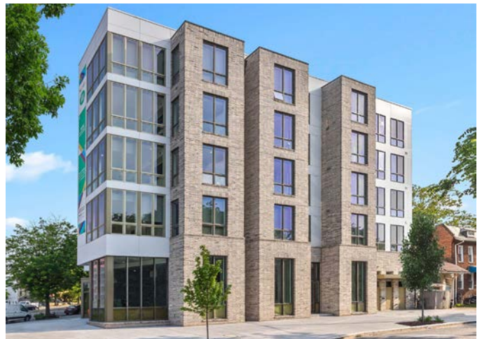
The triangular Modo building in Petworth was designed with entirely three-bedroom, 2-bathroom units. Of the building's 17 units, two are IZ. Source: Communitythree.com.
