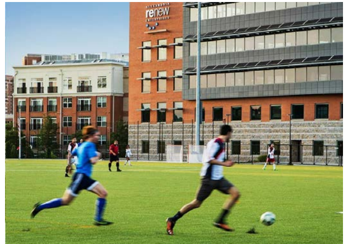
AlexRenew includes a county-run recreational field on the roof of a large wastewater treatment center in Alexandria, VA. Source: Landdesign.com
