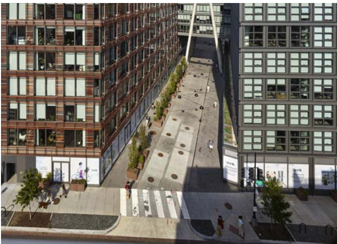
A shared street on private property at the Atlantic Plumbing 091W / Whyte building in DC. Source: ma.com
