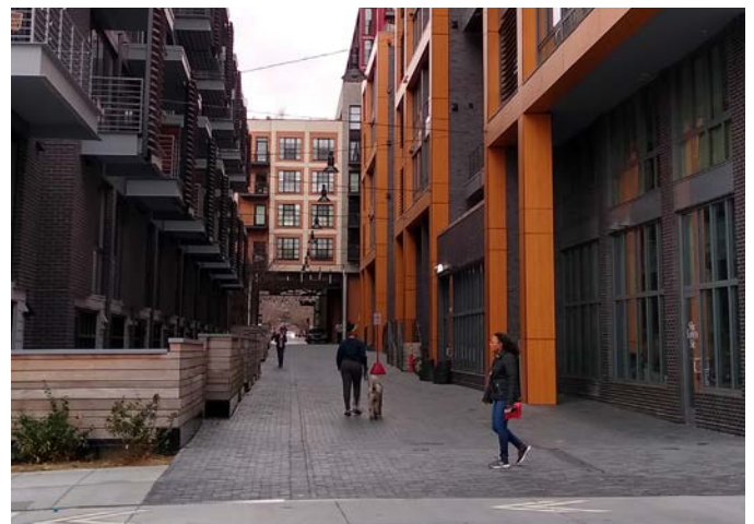
The private shared street in Eckington Yards in DC includes multiple residential and commercial entrances, a loading area, and a small plaza framed by retail.
