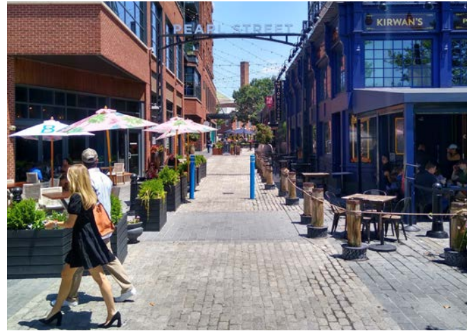
Buildings framing the pedestrian-only Pearl Street at the DC Wharf create a view terminus of the Jefferson Middle School chimney, emphasizing sense of place for the new development.
