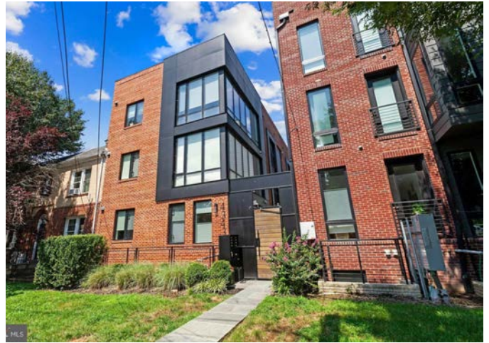
Conversions of four-unit flats on Harrison Street increase the number of for-sale homes in Friendship Heights with two to four bedroom units, but each building contains fewer than 10 units and do not trigger IZ. Source: Compass.com.
