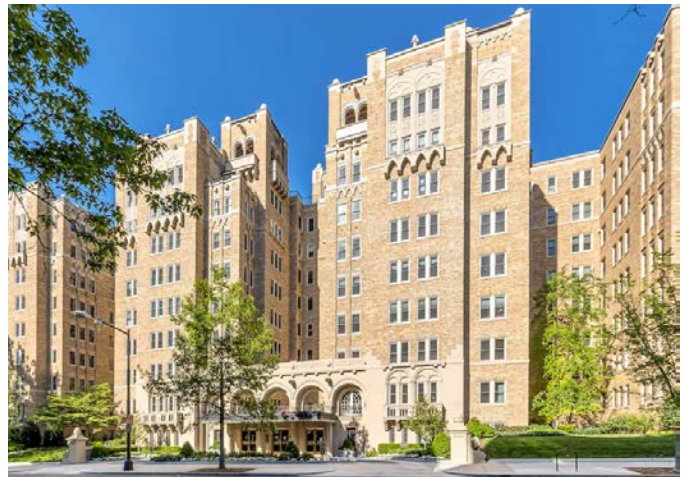
The articulated massing of 2101 Connecticut Avenue allows for each of the building's large 64 units to have light on three exposures. Source: washingtonpost.com.
