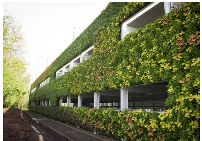
A living green wall could be employed on the southern and 45th street façades of the garage, like this one in Warwick, UK. Source: Archello.com
