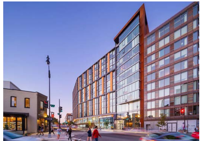
The Wren on Florida Avenue is a prominent apartment building with a grocery store at ground level. Source: hcm2.com.
