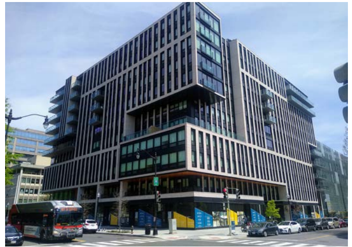
The building massing of 555 E Street SW is articulated with both horizontal and vertical breaks, accommodating balconies and terraces at various levels.
