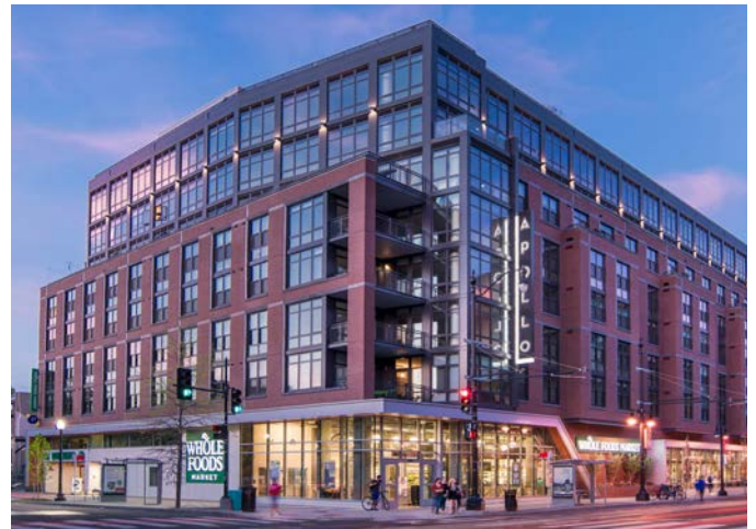
The 431-unit Apollo Apartments on H Street NE includes 25 three-bedroom units (6%), more than is typical for multifamily buildings in DC. The larger units are intended to attract both empty nesters and families. Source: skiarch.com.
