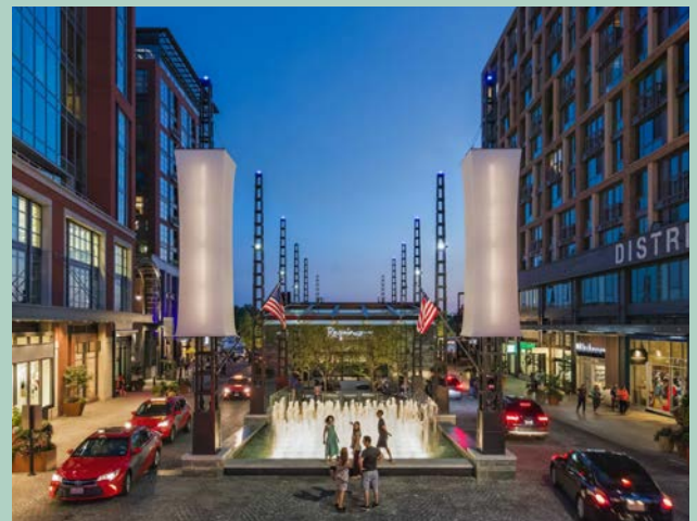
District Square is part of a curbsless shared street network at the Wharf in DC that accommodates people walking and biking, trucks unloading, cars picking up and dropping off passengers, and even outdoor dining. Source: perkinseastman.com.
