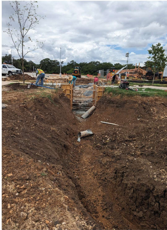
New Trail Head w/ Parking in construction
