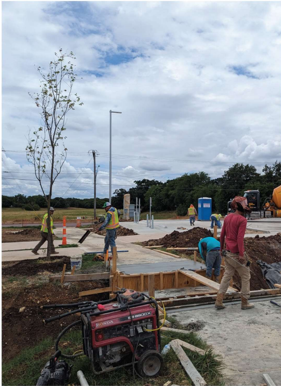
New Trail Head w/ Parking in construction
