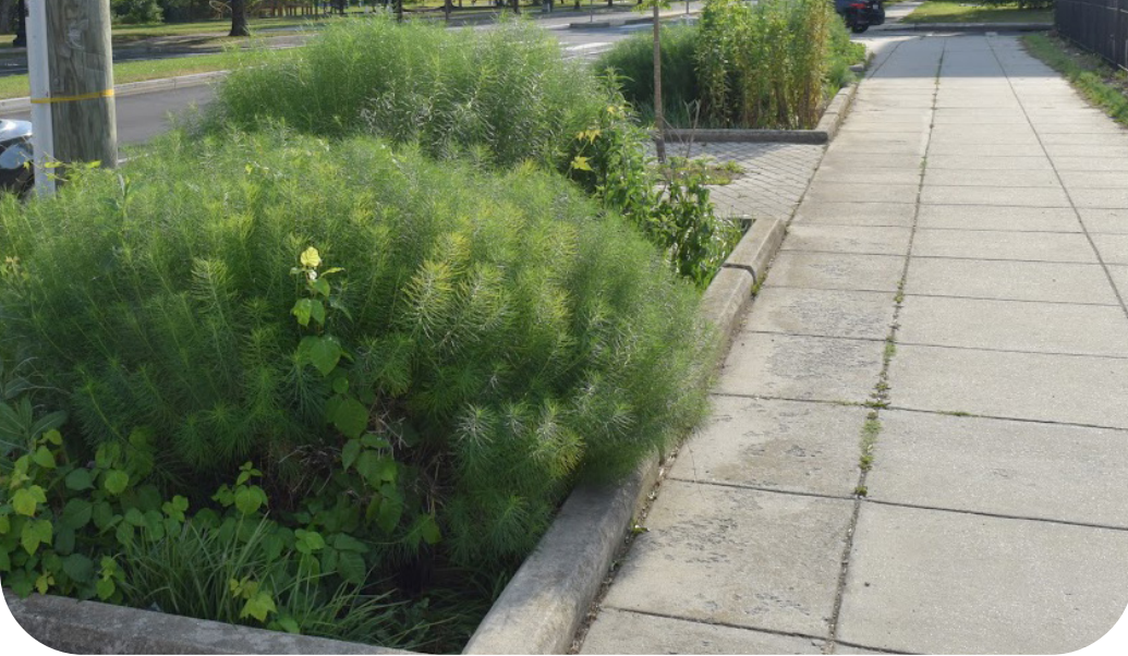
Example of streetscape with green infrastructure elements that reduce stormwater runoff.
