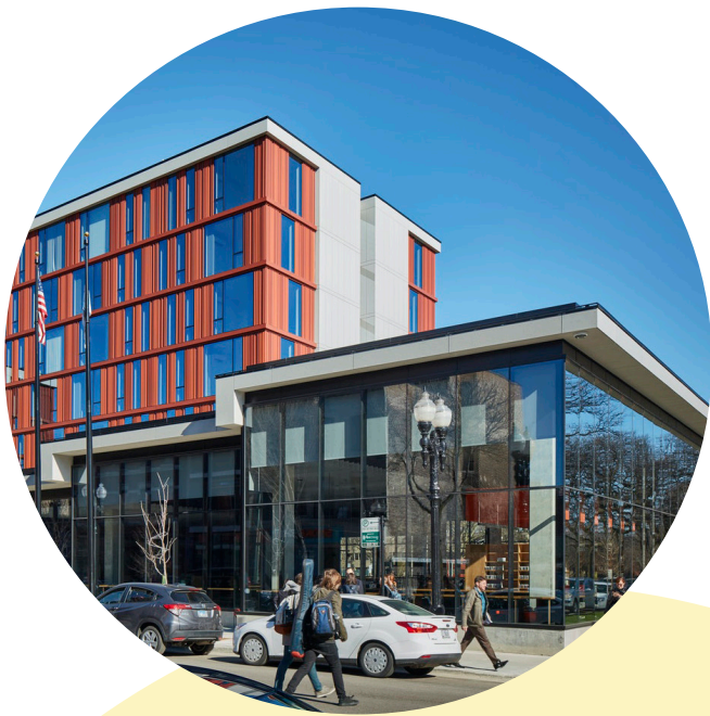
Chicago's Little Italy Branch Library is co-located with mixed-income housing.
