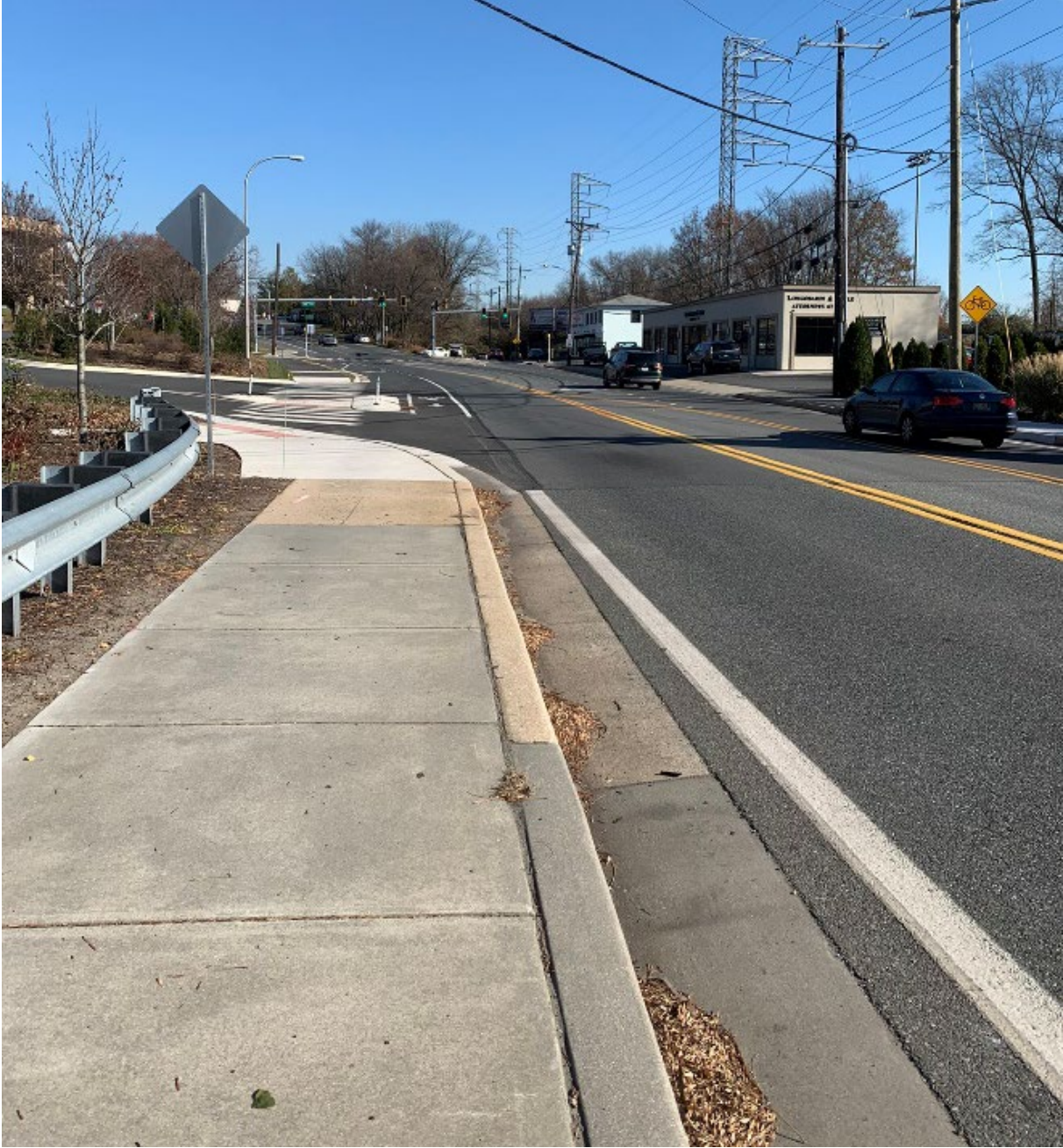
Figure 25. Northeast end of Augustine Cut Off Bridge, looking northeast (towards 18th Street intersection)
