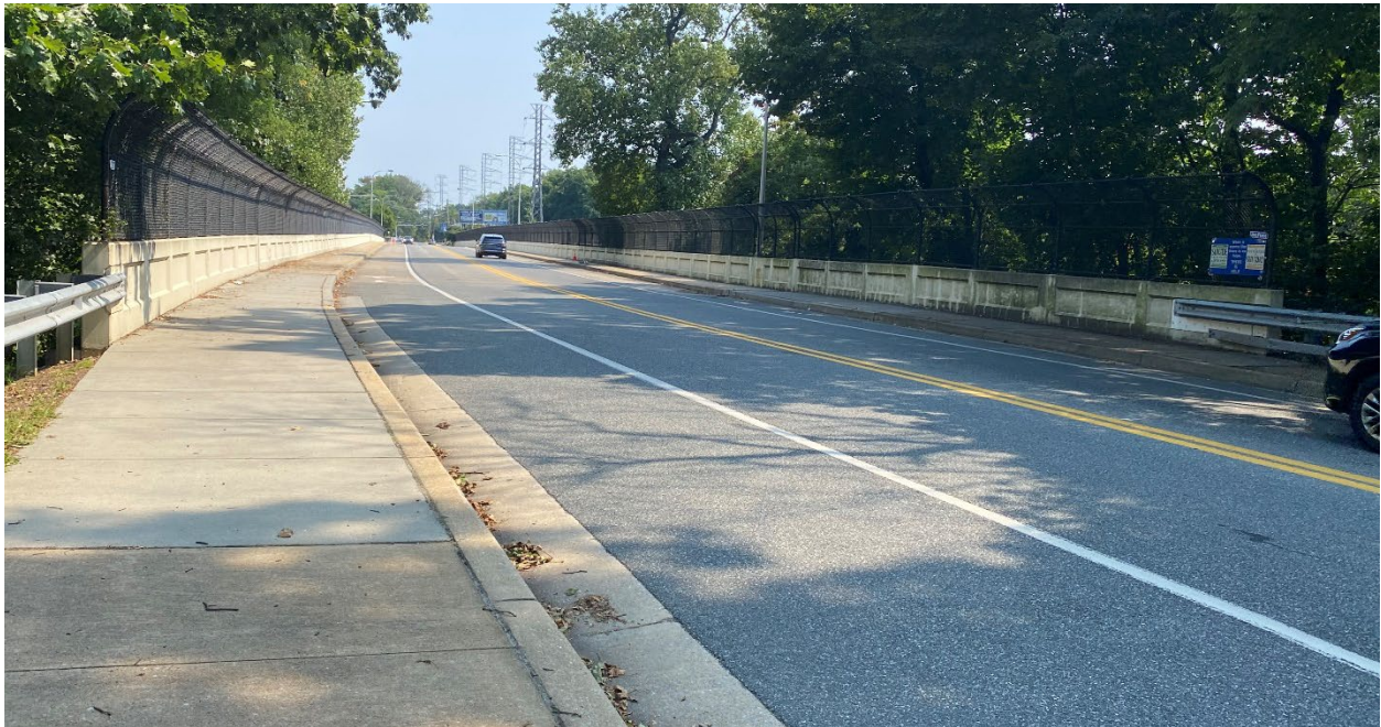
Figure 23. Southwest end of Augustine Cut Off Bridge, looking northeast
