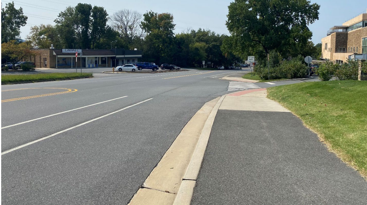
Figure 28. Southbound side of Augustine Cut Off, looking south (towards Stone Hill Road intersection)
