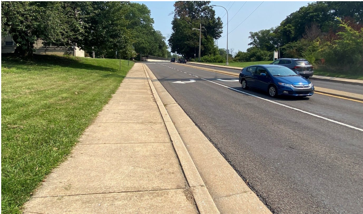
Figure 20. Augustine Cut Off at Lovering Avenue, looking northeast (towards Wawaset Street)
