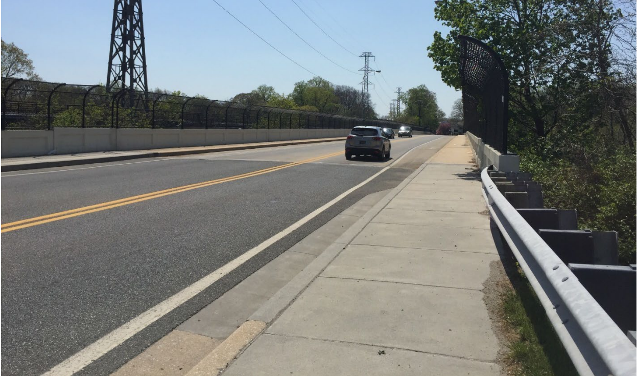
Figure 24. Northeast end of Augustine Cut Off Bridge, looking southwest
