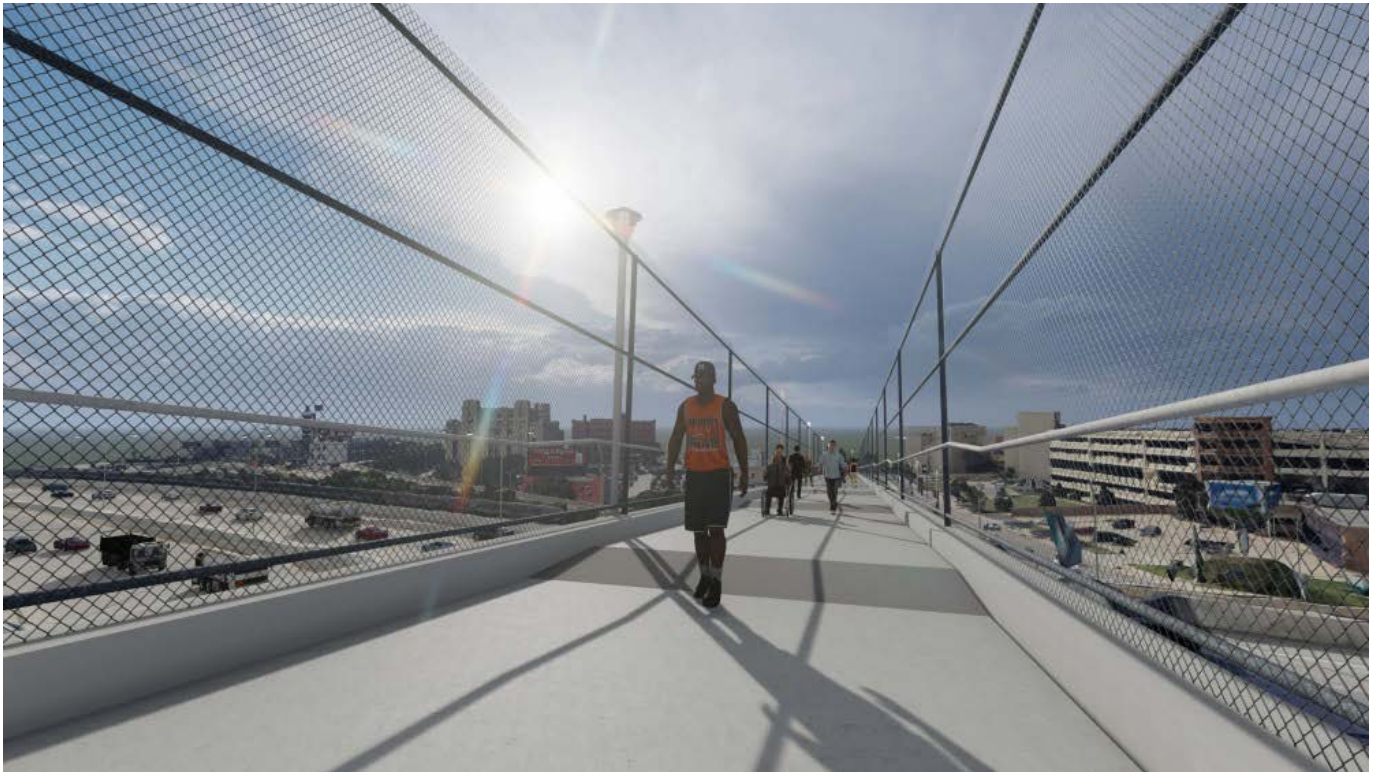
Views of the Alternative 1 bridge deck looking down toward downtown. The darker areas of pavement are flat respite areas that are five feet in length. (Click image to enlarge)
