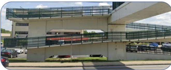
Concrete Slab Ramp
