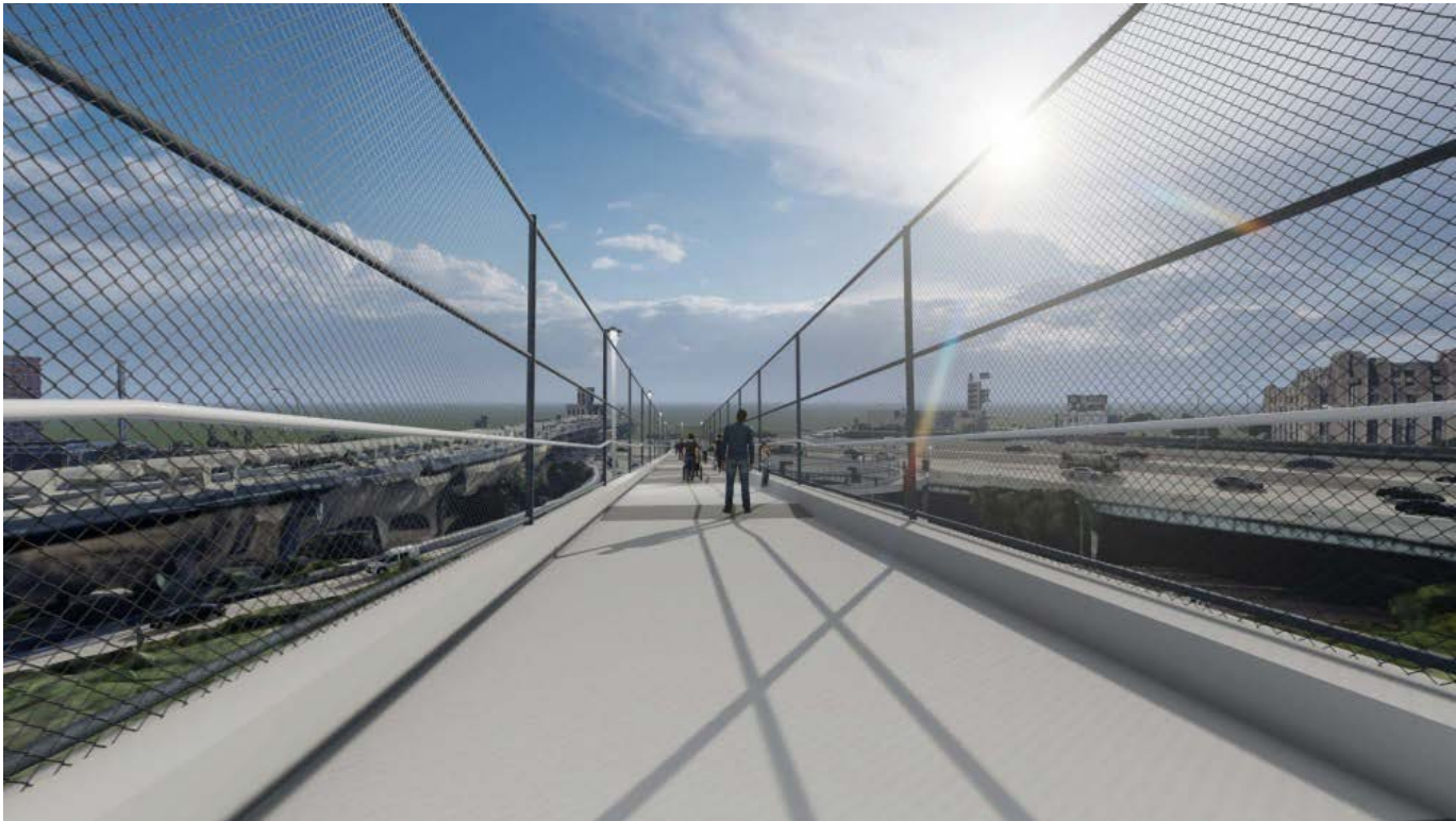
View of the Alternative 2 looking toward downtown. The darker areas of the bridge deck are flat respite areas that are five feet in length. (Click image to enlarge)
