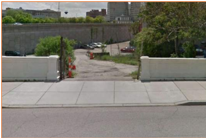
Photo 5 - 1 E. Court St. Parking Entrance
