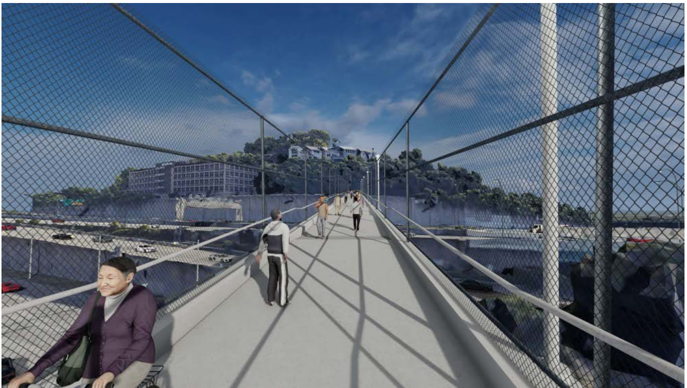
Views of the Alternative 1 bridge deck looking up toward Mt. Adams. The darker areas of pavement are flat respite areas that are five feet in length. (Click image to enlarge)
