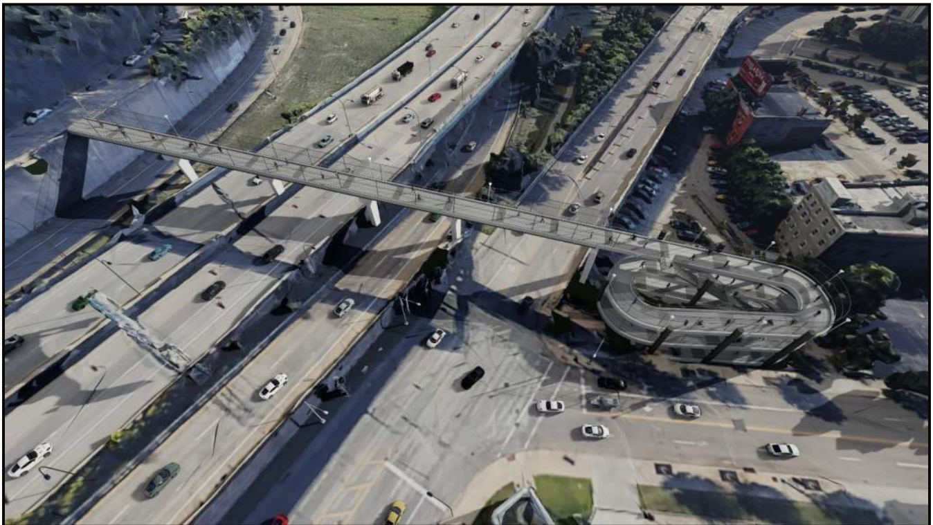
Figure 1-1 Alternate 1: Aerial view looking south.
