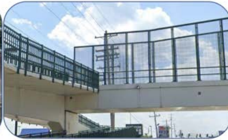
Concrete Box Beam
