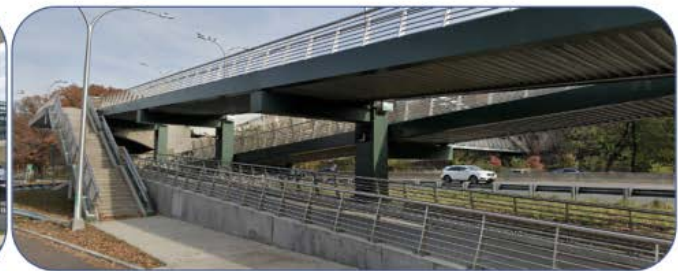
Steel Beam Ramp
