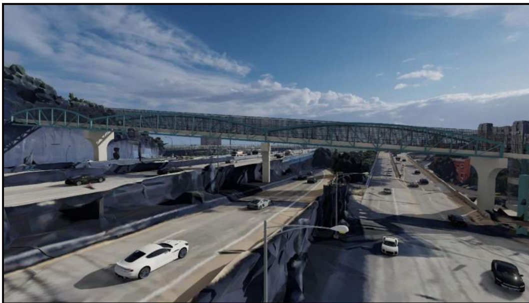
Figure 7-1 Preferred Alternate: View looking south.
