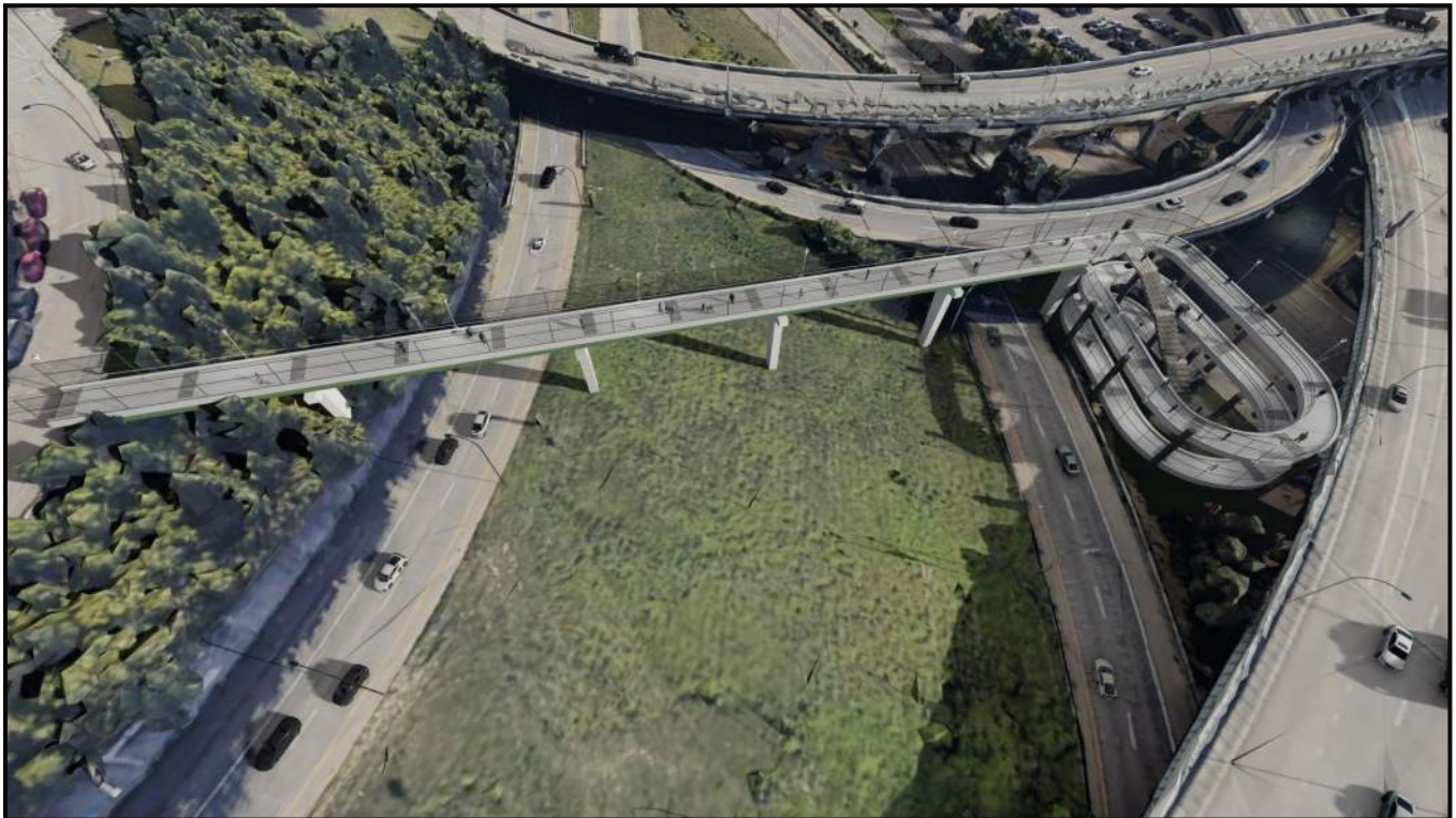
Figure 2-1 Alternate 2: Aerial view looking south.
