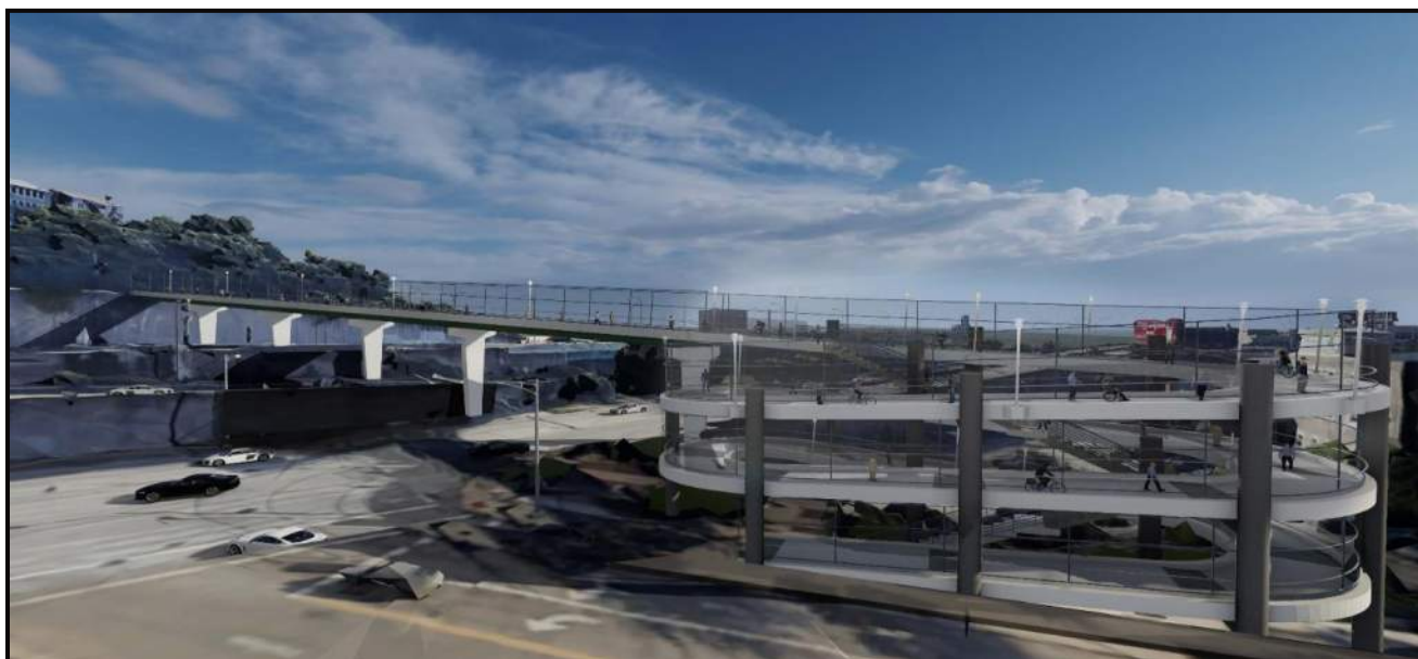
Figure 1-2 Alternate 1: Looking south at ramp structure.
