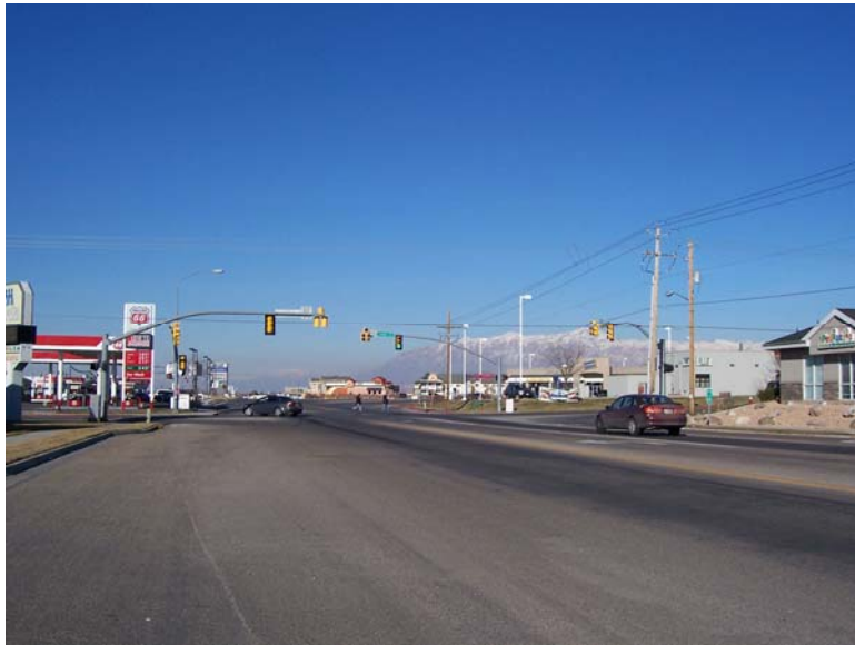
Photo 3.16-1. S.R. 108 and 4800 South Intersection Looking South
