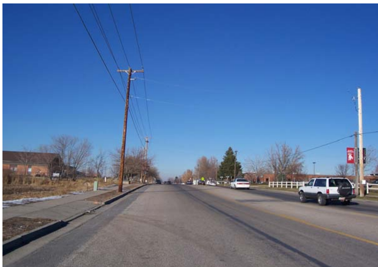
Photo 3.16-4. S.R. 108 in Syracuse near Syracuse Elementary School and Syracuse Junior High School Looking North
