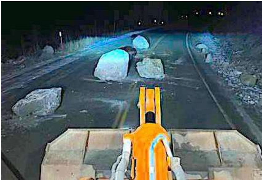
Boulders on the Long Lake Hill in the highway driving lanes. These create extreme danger at night with already limited visibility from the road curves and steep hill. There is also no maneuvering room. If there is oncoming traffic, there is no shoulder and a steep cliff up or down depending on which side you end up going off.
