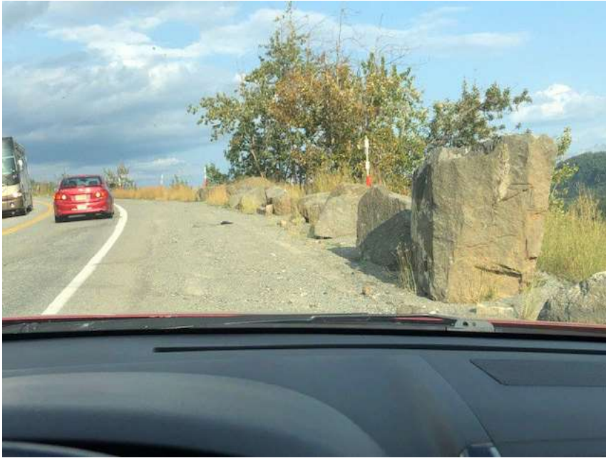
Boulders on Long Lake Hill. These land on the road, and sometimes on vehicles and present severe limited visibility hazards until they are pushed to the side of the road.
