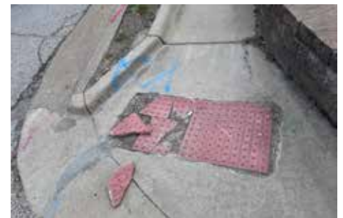
Broken ADA detectable warning device on Rainbow
