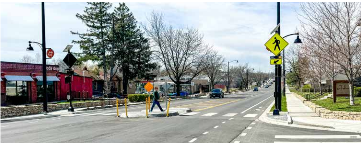
Figure 67. Pedestrian Median Refuge Island with Rectangular Rapid Flashing Beacons on 47th Ave.
