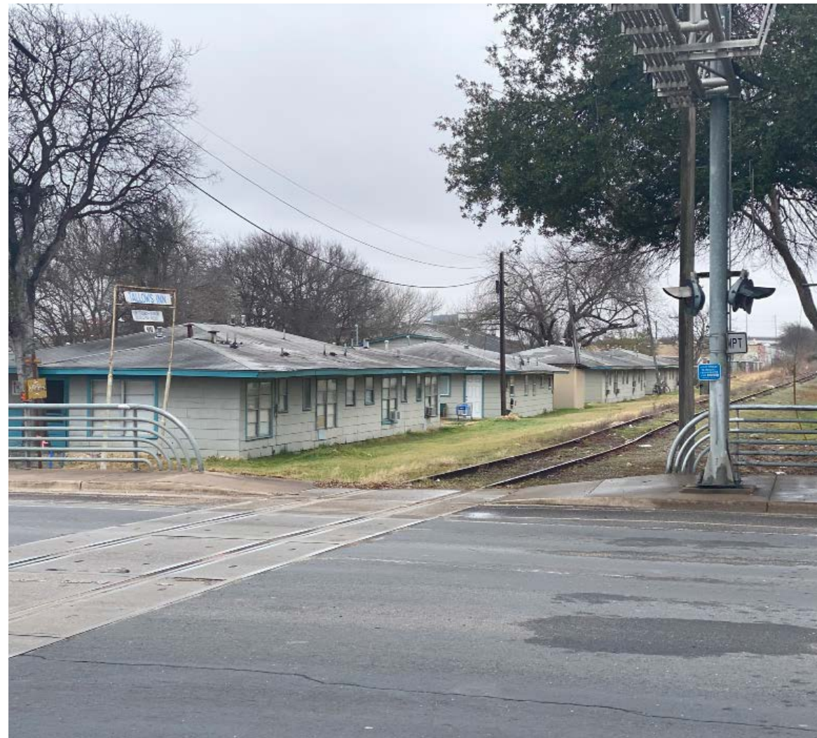
Rail crossing at South Congress which is part of the planned Bergstrom Spur Trail
