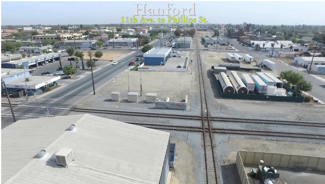
Figure 6-17: Hanford at the BNSF railroad crossing, looking east
