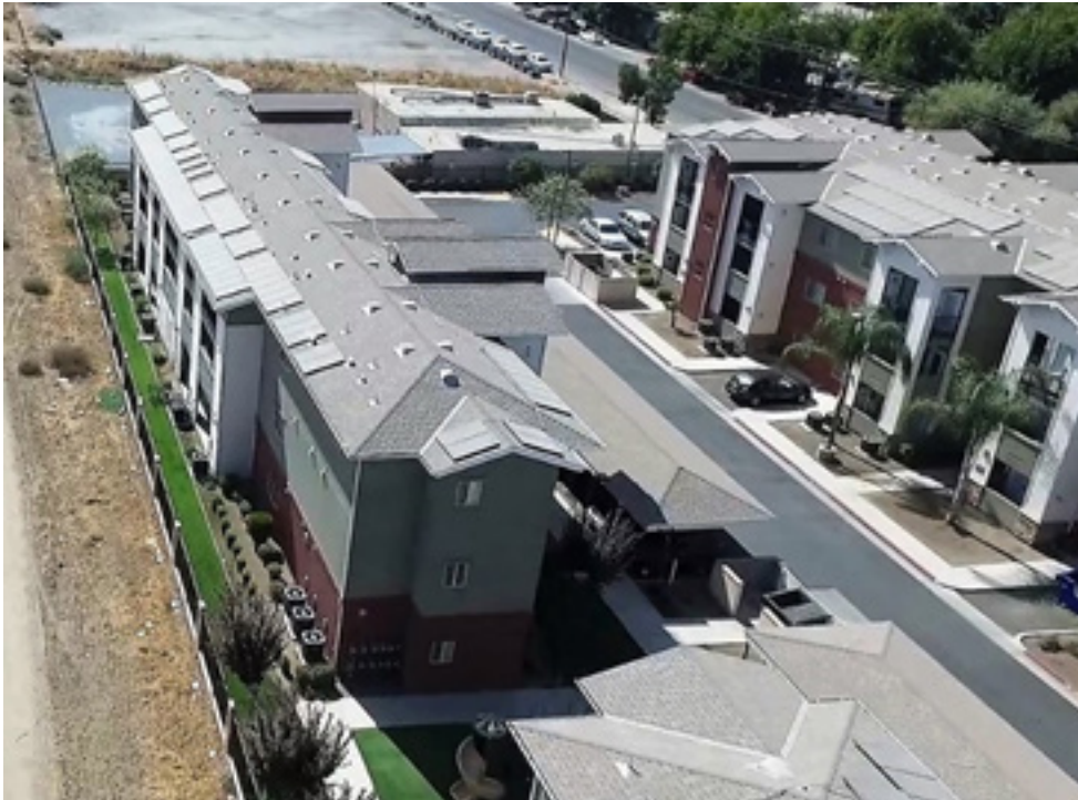
Figure 6-3: Multi-family housing near the Cross Valley Corridor in Porterville
