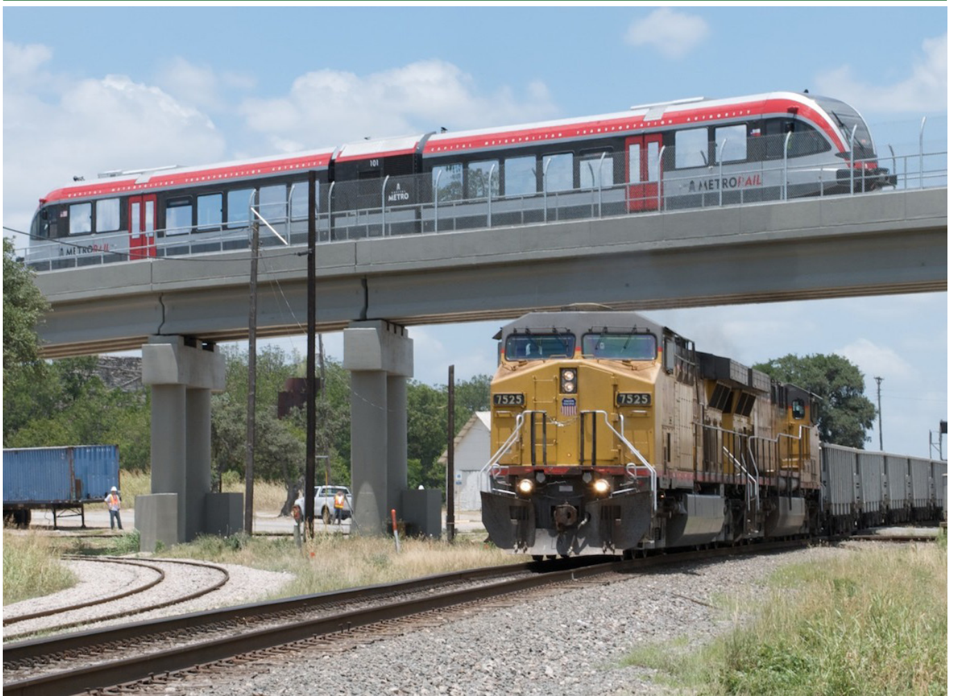
Figure 4-1: A Capital MetroRail DMU Train in Austin, Texas
