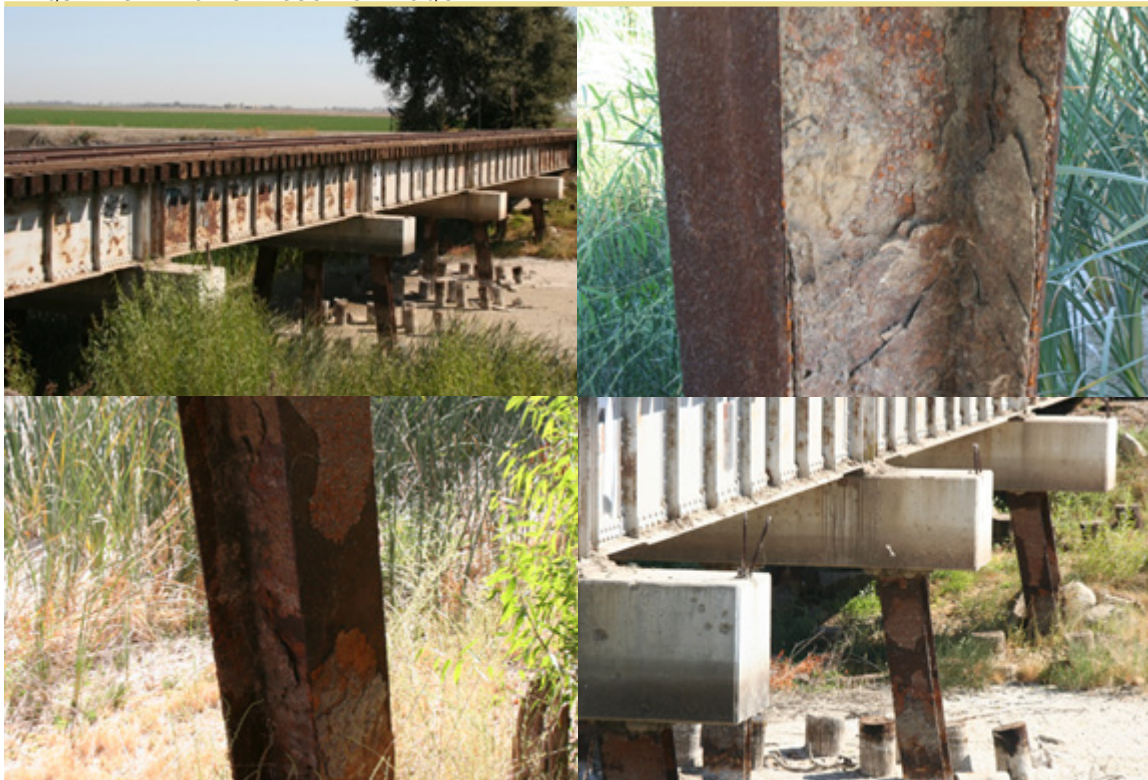
Kinas River Wildlife Preserve Bridge
