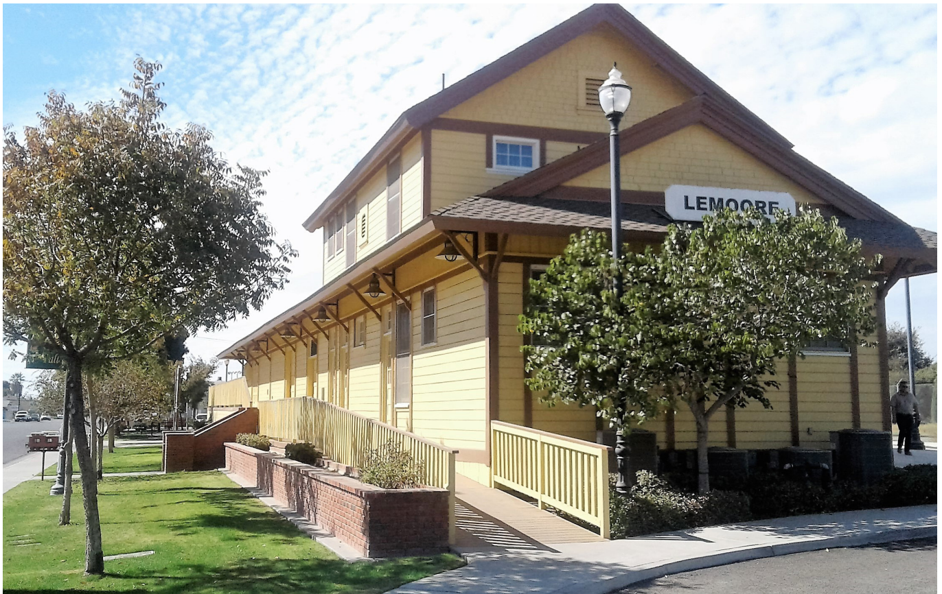
The Depot is a good example of symbolic architecture that can serve as one of the City’s more identifiable and memorable landmarks for a Cross Valley Corridor station
