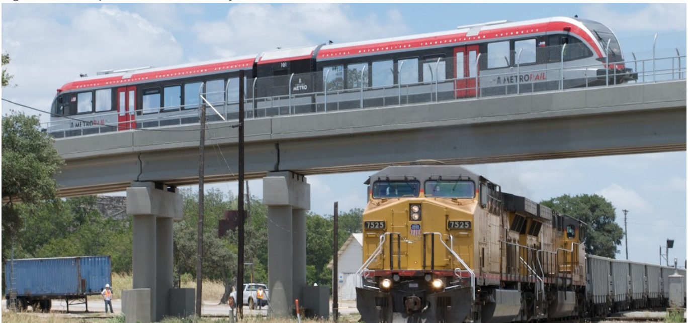
Figure ES-18: Capital MetroRail DMU System in Austin, Texas
