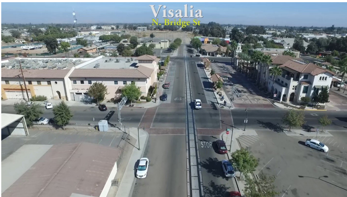
Figure 6-21: The Visalia Transit Center, looking east
