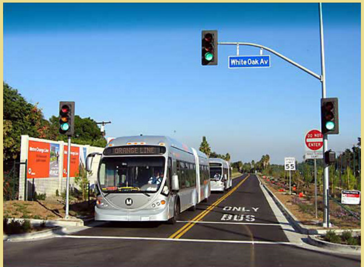
Figure ES-14: Los Angeles Metro Orange Line Bus Rapid Transit - Dedicated Bus Lane
