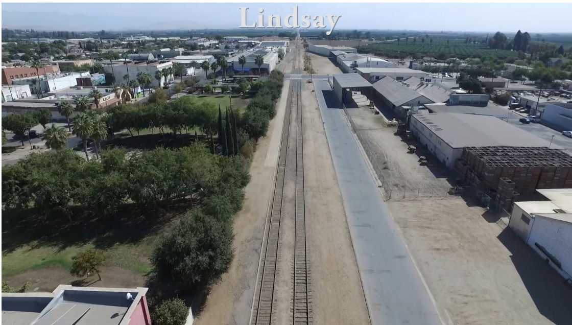
Figure 6-33: Lindsay station area, looking south
