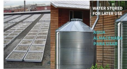
Collecting water from roofs and other surfaces Recolectar agua de techos y otras superficies
