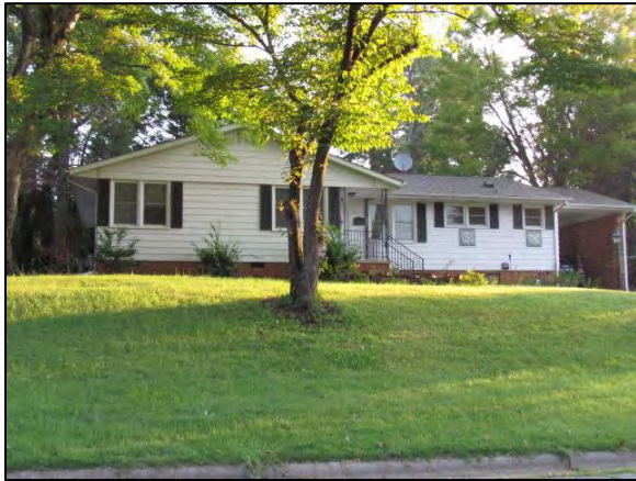
Figure 63: Clockwise from upper left, 913 Onslow Drive, 2802 New Hanover Drive, and 2510 Fairway Drive are cross-gable Ranches with rectangular massing and feature minimal simple details. 913 Onslow and 2802 New Hanover Drive have minimally recessed front entrances. 913 Onslow has three different window sizes while 2802 New Hanover Drive has asymmetrically placed sets of tall casements windows. 2510 Fairway Drive, ca. 1960 features a brick screen at the carport and a deeper recessed entrance.
