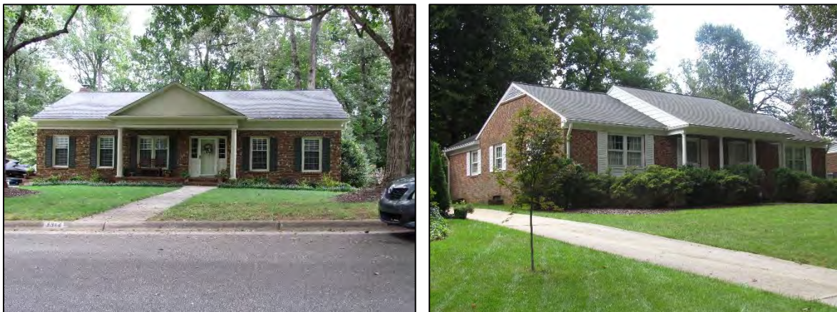
Figure 65: from L to R: 3312 Northampton Drive and 1202 McDowell Drive represent Ranch forms with Colonial Revival details. The typical Colonial Revival-style details found on Ranches in Green Valley are an over scaled pedimented porch centered on the width of the house or a fully engaged portico, also centered. Colonial Revival-style ranches have near symmetrical fenestration and massing and consistently feature the same window width equally spaced on the front elevation.
