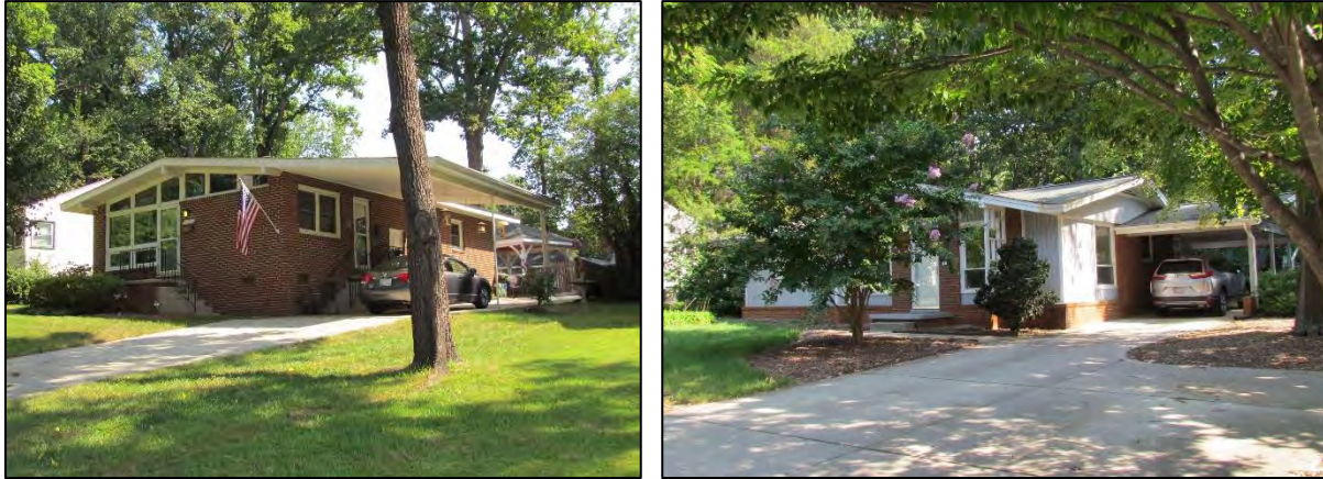
Figure 54: L to R, 2703 Evergreen Drive features a low-pitched gabled roof with clerestory windows and 2712 Shady Lawn Drive displays a butterfly roof and mix of façade materials.
