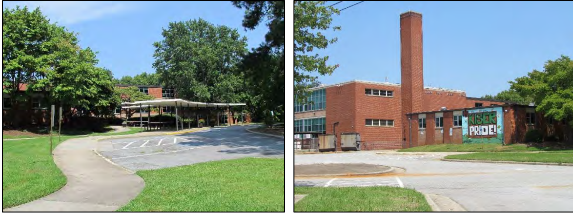
Figure 24: L to R, the covered walkway leading to the main entrance and view of Buildings 1 and 2
