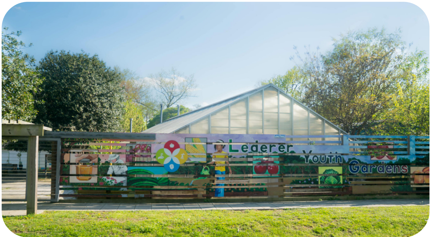
Lederer Gardens is a community garden serving surrounding residents and visitors. Its location directly on Nannie Helen Burroughs Avenue represents the potential for public space activation connecting park green space to the town square concept.
