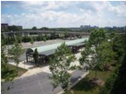
Bottom: Office building and Wetlands in the Herndon District TOD
