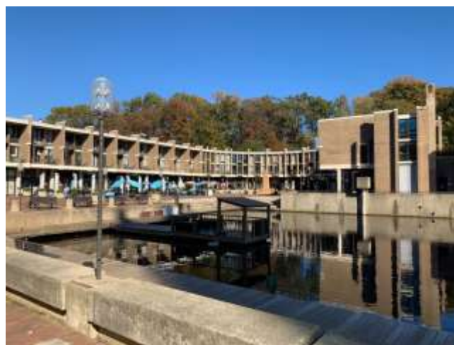
Below: Historic Lake Anne Village Center
