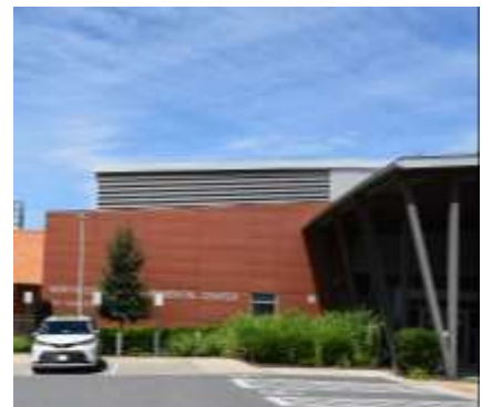
Below bottom: Bioswale
