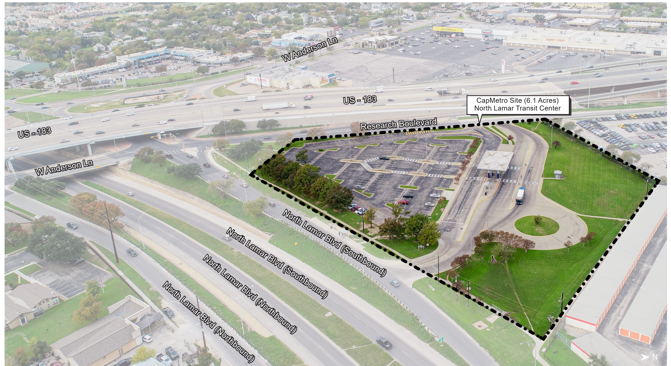
Figure 11: North Lamar Transit Center aerial
