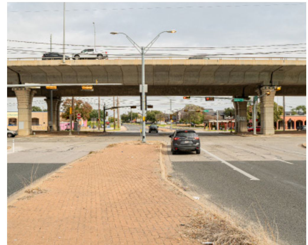
Disconnected sidewalks and intrusive infrastructure
