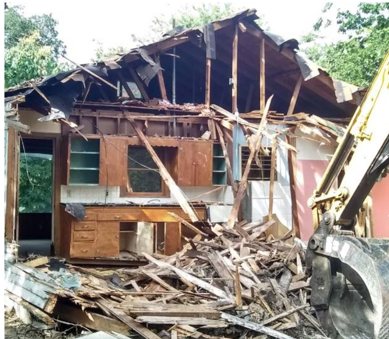
▲ Older home during demolition
