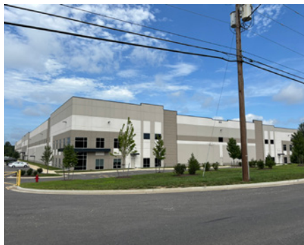
Route 1. Newer distribution/warehousing development
