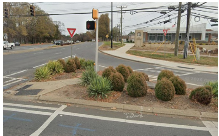
Intersection landscaping and safety improvements
