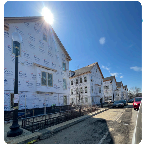
Townhouses under construction at St. Elizabeths
