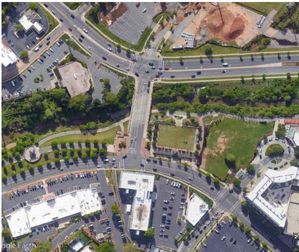
3.8 Unearthing the stream provided space for the greenway trail and reconnected the creek to its watershed.
