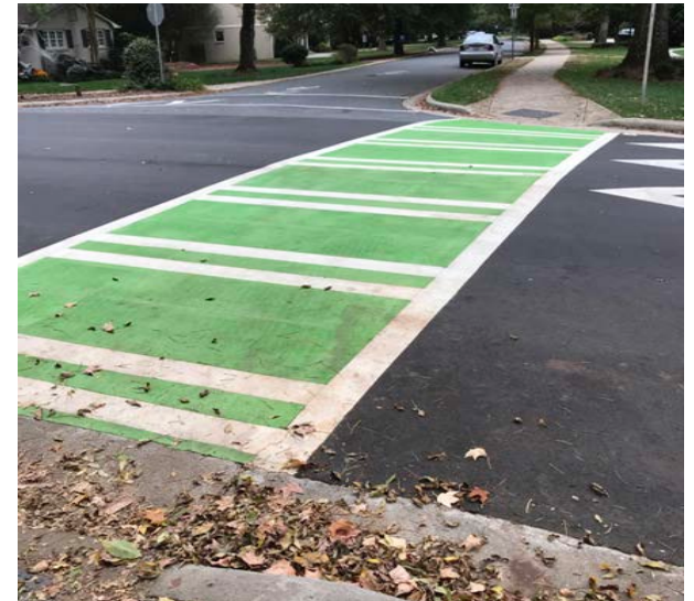
5.20 Colored crosswalks can improve safety at road crossings. This particular example displays the City's urban trail standard.
