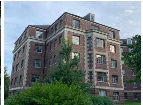
South Cathedral Mansions - Multi-story large residential complex
