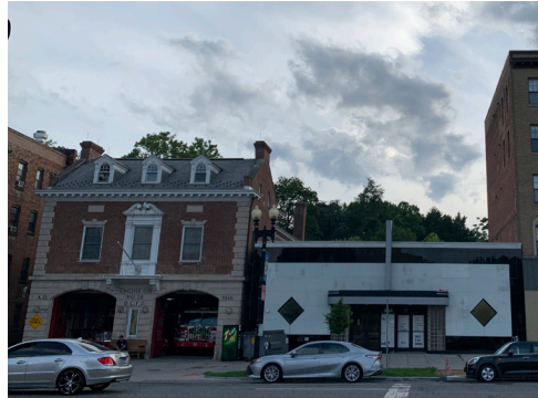
Fire Station & art deco commercial near corner of Porter St.
