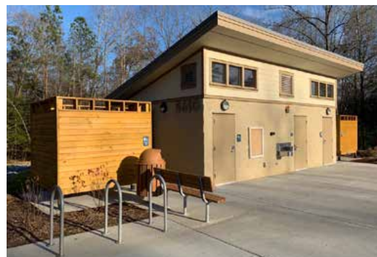
Existing Comfort Station & Changing Rooms
