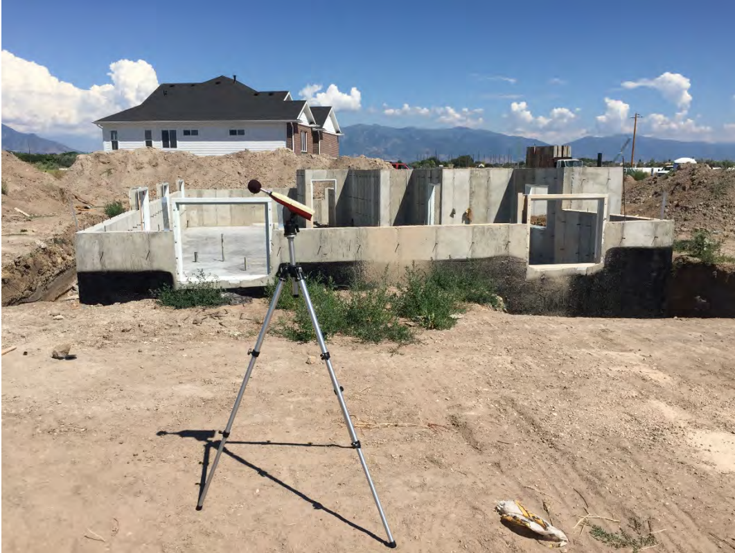
Site 2. Looking East
