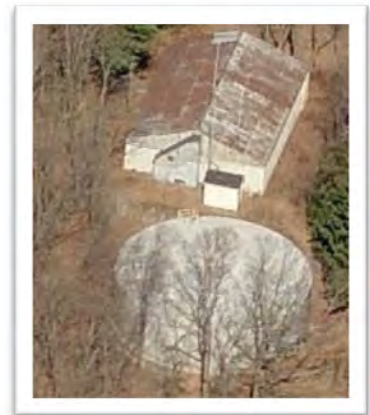
Photo 14-1: Water tank in Essex Fells
