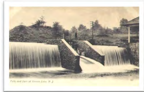
Photo 9: Dam at Lake Verona
