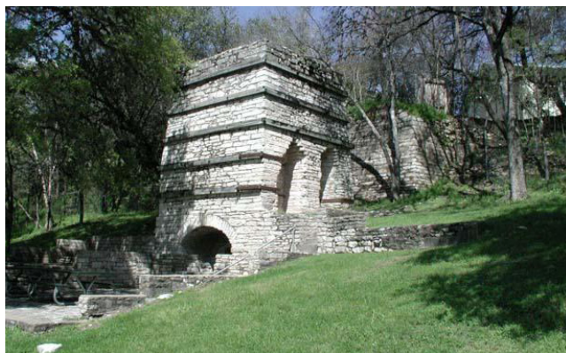
▲ The Taylor Lime Kiln in Reed Park was built in 1871 to manufacture lime from local limestone. The site has multiple well-preserved features that tell the story of how the kiln worked.
