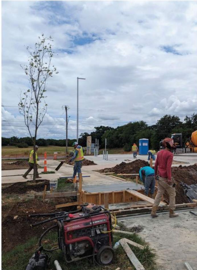
New Trail Head w/ Parking in construction
