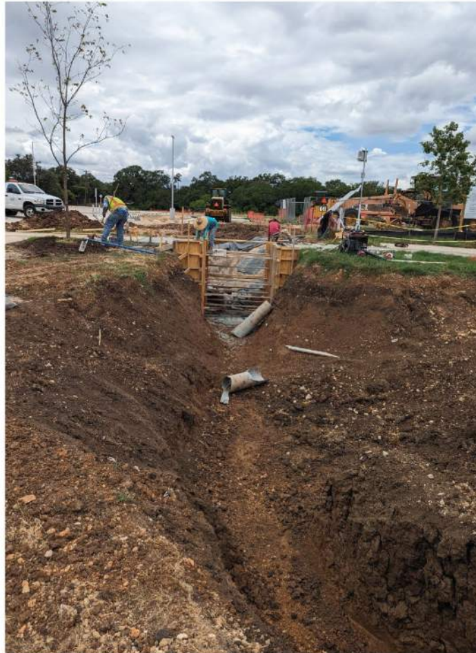
New Trail Head w/ Parking in construction
