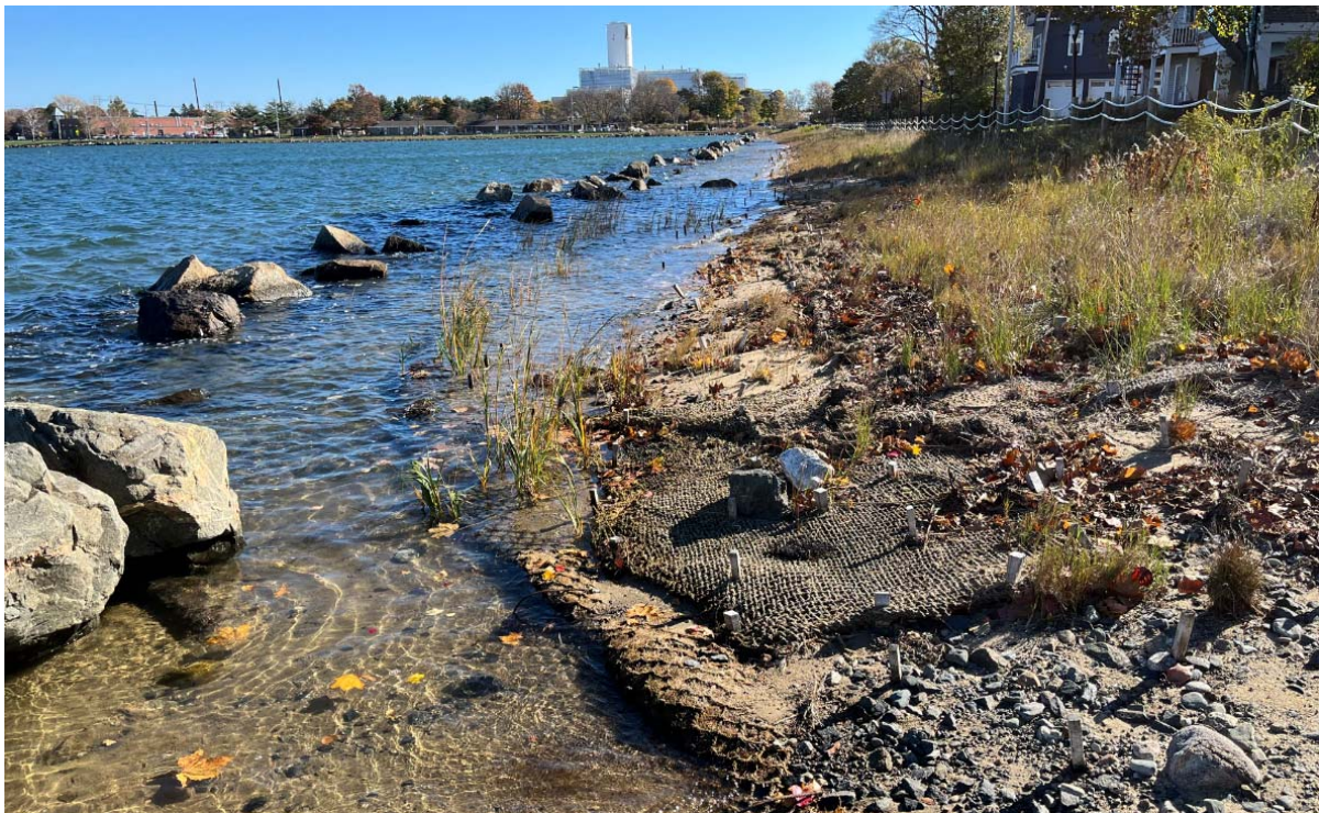
Figure 9. Example of a Natural Shore Protection Structure in the Study Area (December 2022)
