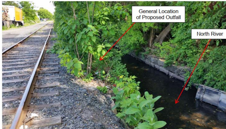
Figure 12. The North River, to which Stormwater will be Discharged via the New Drainage Pipe (Shown Above). Stormwater is collected by a series of catch basins and drains to the north river via one existing outfall. Image Source: AECOM.
