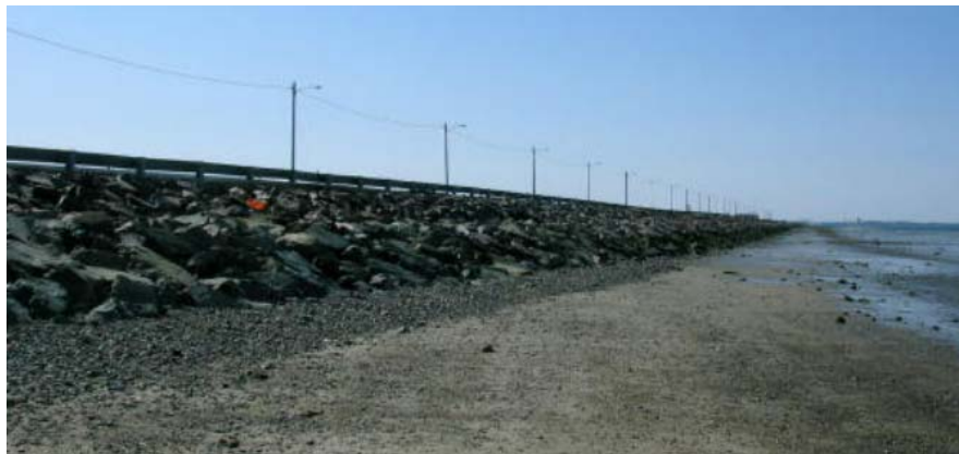
Figure 21. Revetment in Nahant, Massachusetts. Image Source: TenCate Geosynthetics .
