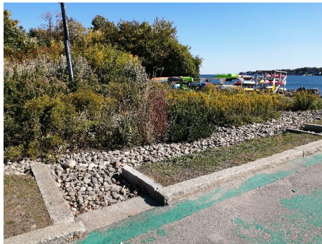
Figure 14. Rain Garden in Salem, Massachusetts. Image Source: Barbara Warren, Salem Sound Coastwatch.
