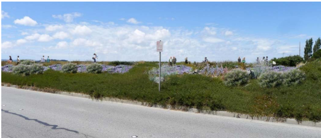
Figure 20. Proposed Earthen Levee in Foster City, California. Image Source: Levee Improvements Project .
