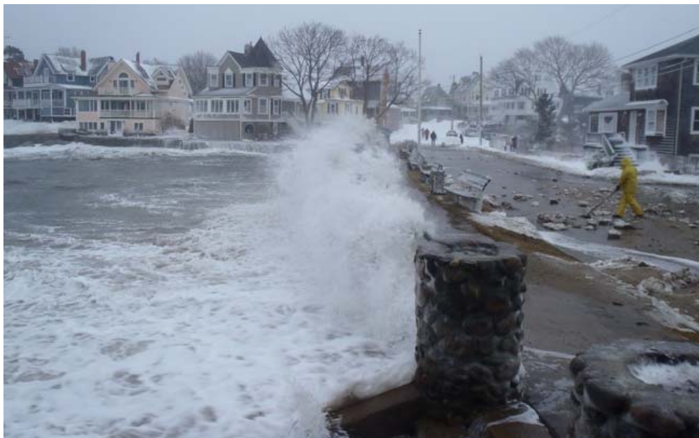
Figure 3. Wave Breaking on Juniper Beach Seawall During a 2013 Nor'easter (Swin, 2013)
