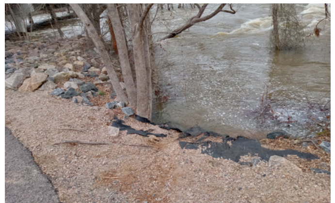
Figure 36: Erosion of the southern tributary and riverbank due to stormwater flow from uphill streets and neighborhoods.
