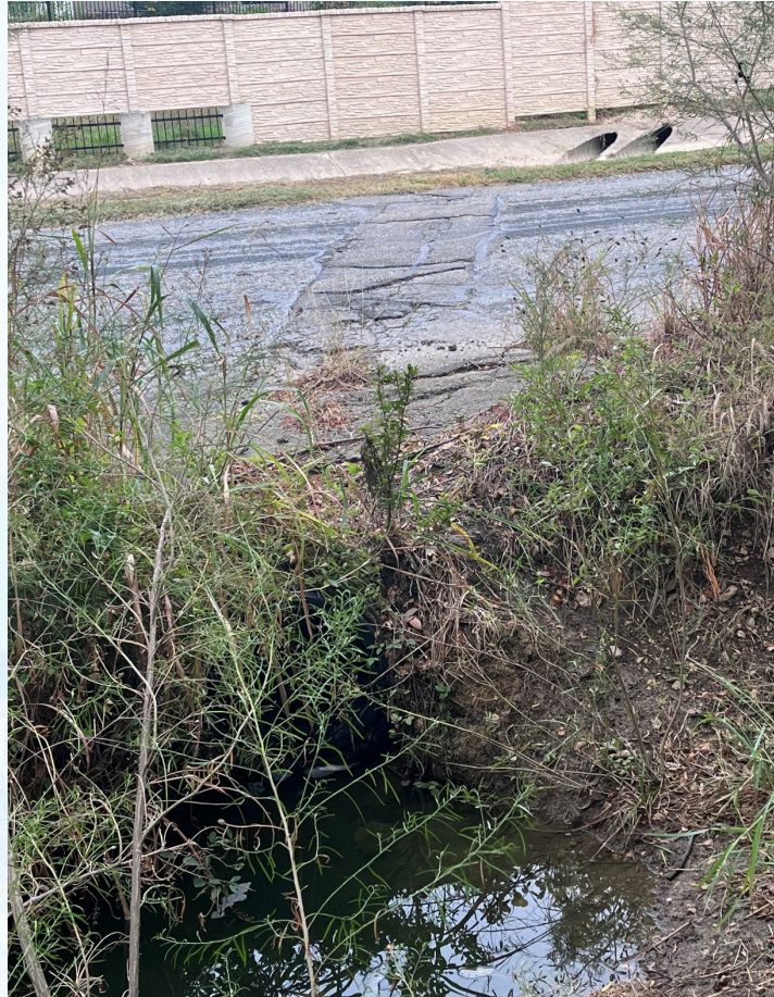
Culvert across Southwell– Facing East
