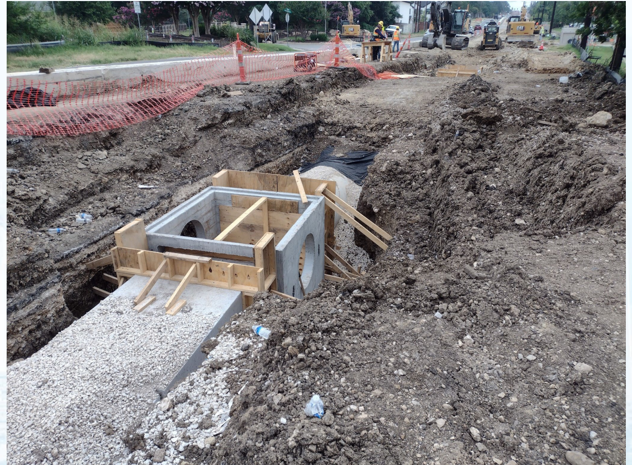
Storm drain installation along Prue Road showing similar underground work.
