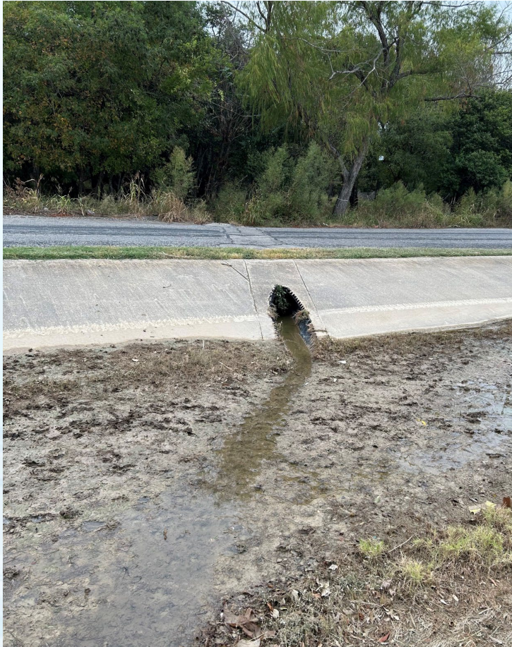
Southwell drainage structure – Facing West
