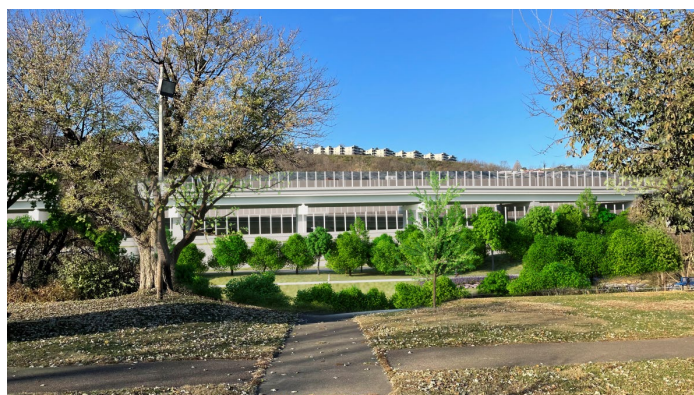
Potential transparent noise barriers near the Goebel Park Complex are being coordinated with the Covington Aesthetics Subcommittee to preserve views of the park from the highway (looking west).
