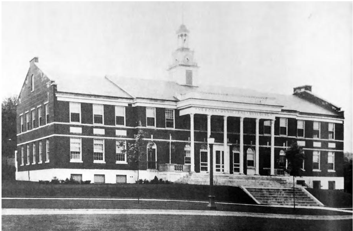
Historic photo shortly after completion
