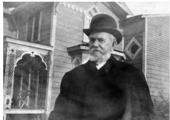
Historic photo of Capt. Cook at the home
