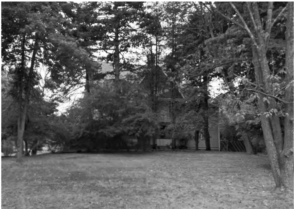
2013 view before demolition
