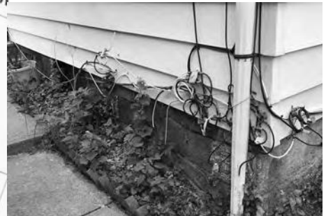
Evidence of dressed sandstone foundation
