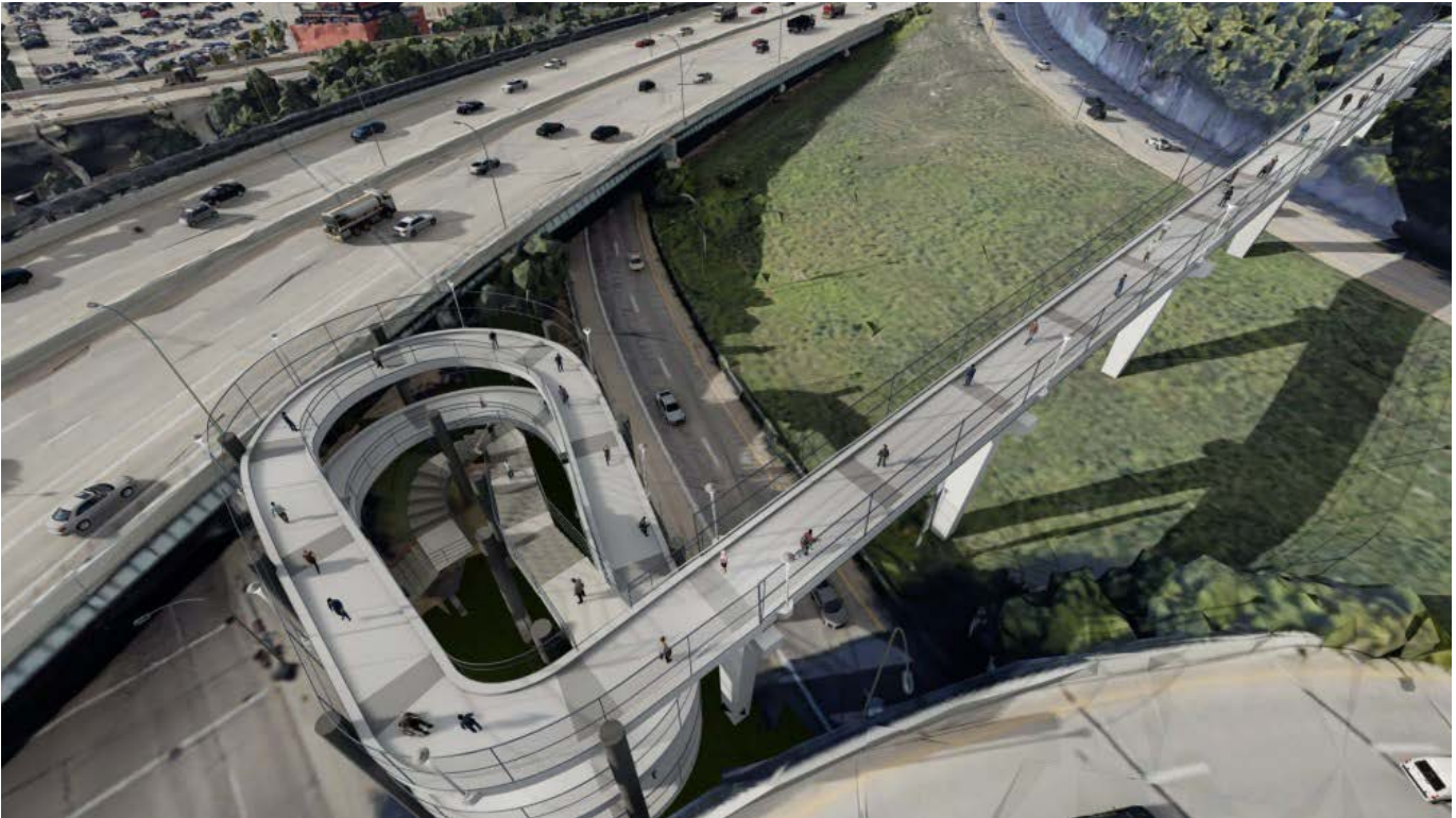
An aerial view of the three-tier ramp and stair system on the west end of Alternative 2. The ramp would be nested in between I-71 and Columbia Parkway/US 50. (Click image to enlarge)
