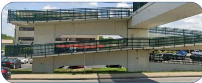
Concrete Slab Ramp
