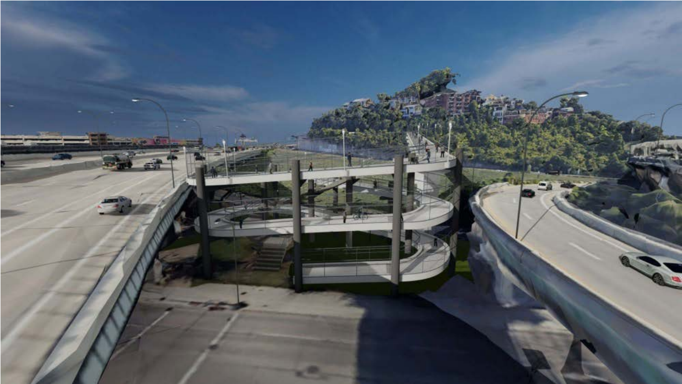
Another view of the three-tier ramp and stair system on the west end of Alternative 2, looking east toward Mt. Adams. The ramp would be nested in between I-71 and Columbia Parkway/US 50. (Click image to enlarge)
