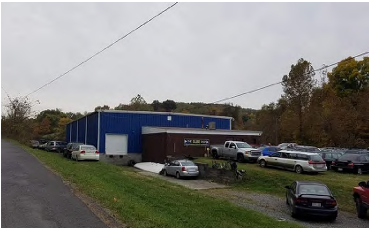
Photograph 2. East and north (front) elevations, facing southwest
