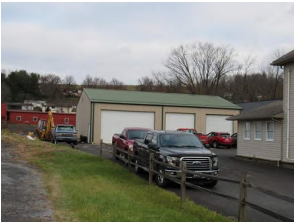
Photograph 2. Garage north of house, facing north (Markosky 2018-12-04)
