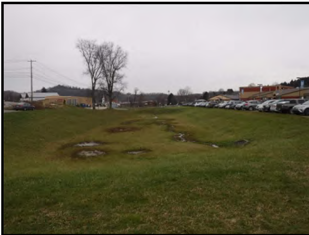
Photograph 40. View of a drainage basin in the study area, facing southwest.
