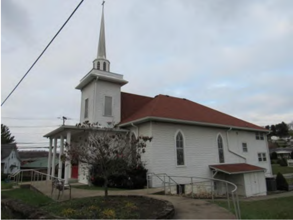
Photograph 1. MG-1332 / Harner Chapel, Morgantown, Monongalia County Northeast elevation, facing northwest
