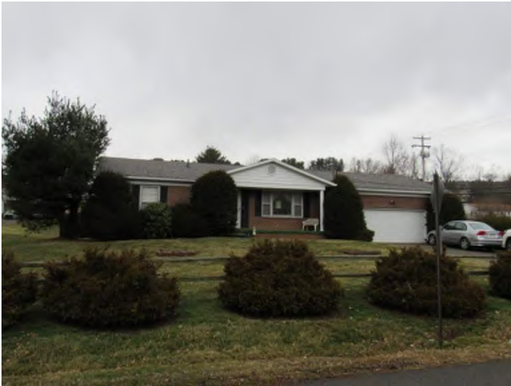
Photograph 1. House and garage, facing north (Markosky 2019-02-05)
