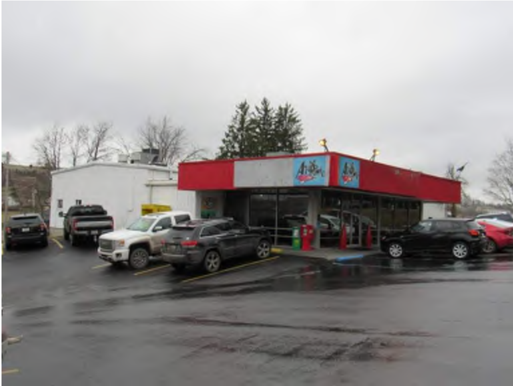
Photograph 1. Main entrance, facing northeast (Markosky 2019-02-05)
