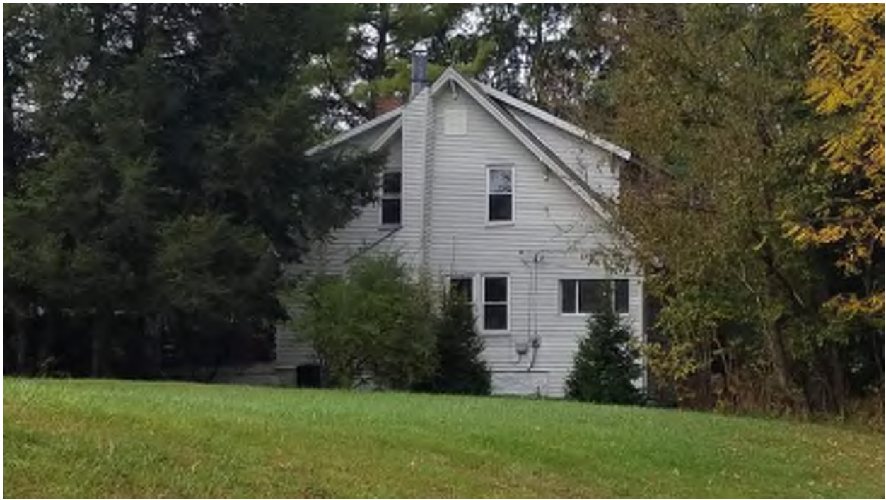
Photograph 1. East (side) elevation, facing west
