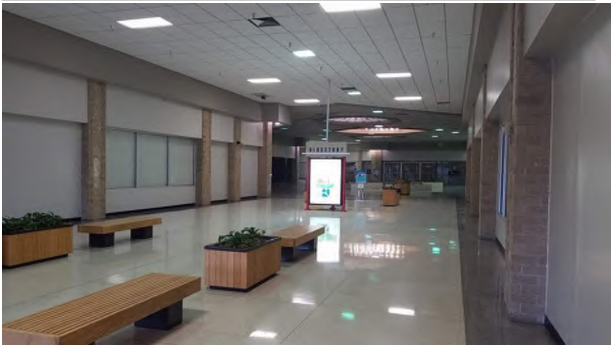
Photograph 7. Terrazzo floor, glazed brick pilasters, and planters (Markosky 2019-03-20)
