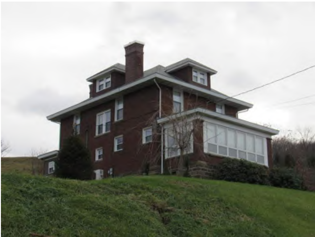
Photograph 2. House showing enclosed front porch, facing southeast (Markosky 2018-12-04)
