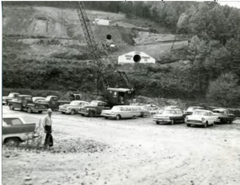
Inset 9. Greenbag Cement Company plant near Greer, Monongalia County, ca. 1961 (WVU 1961a).
