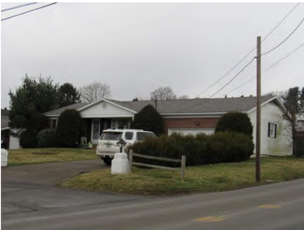
Photograph 2. Façade and northeast elevation, facing northwest (Markosky 2019-02-05)
