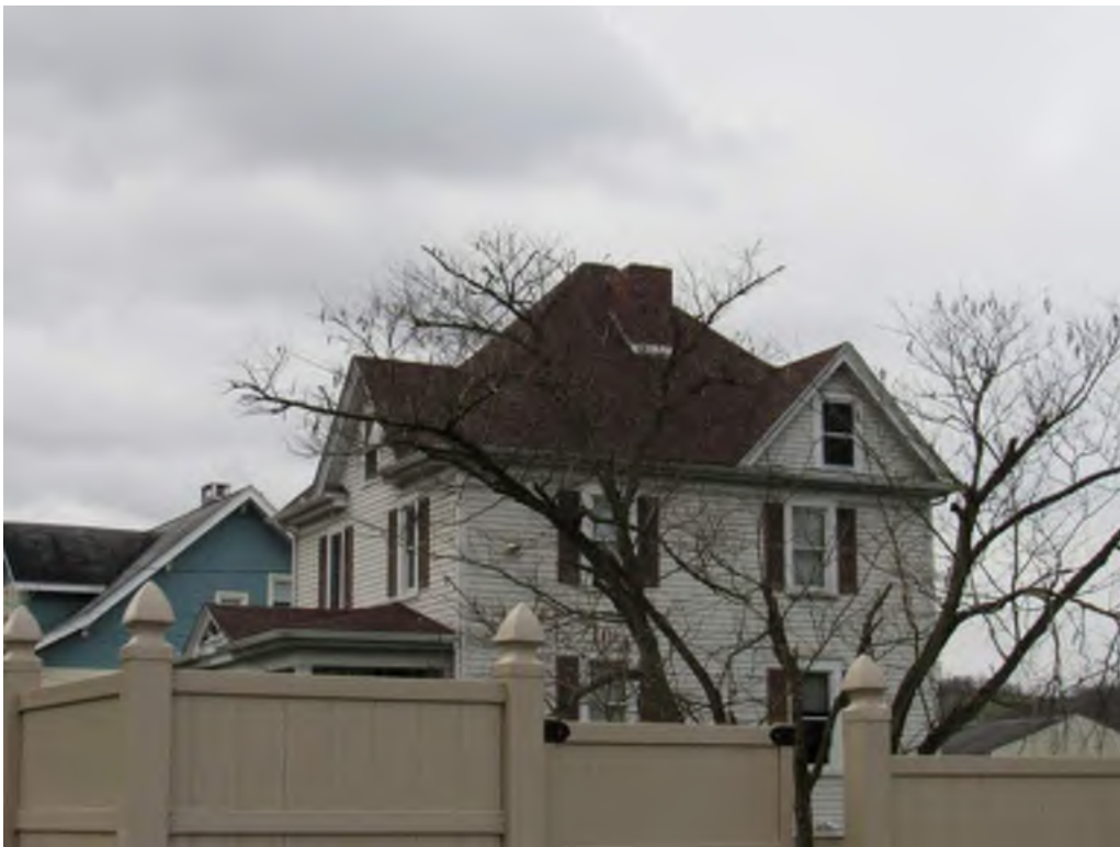
Photograph 2. East and north elevations, facing southwest (Markosky 2018-12-04)
