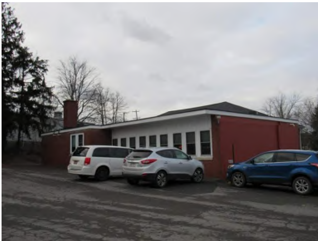
Photograph 2. Rear addition, facing southwest (2018-12-05)
