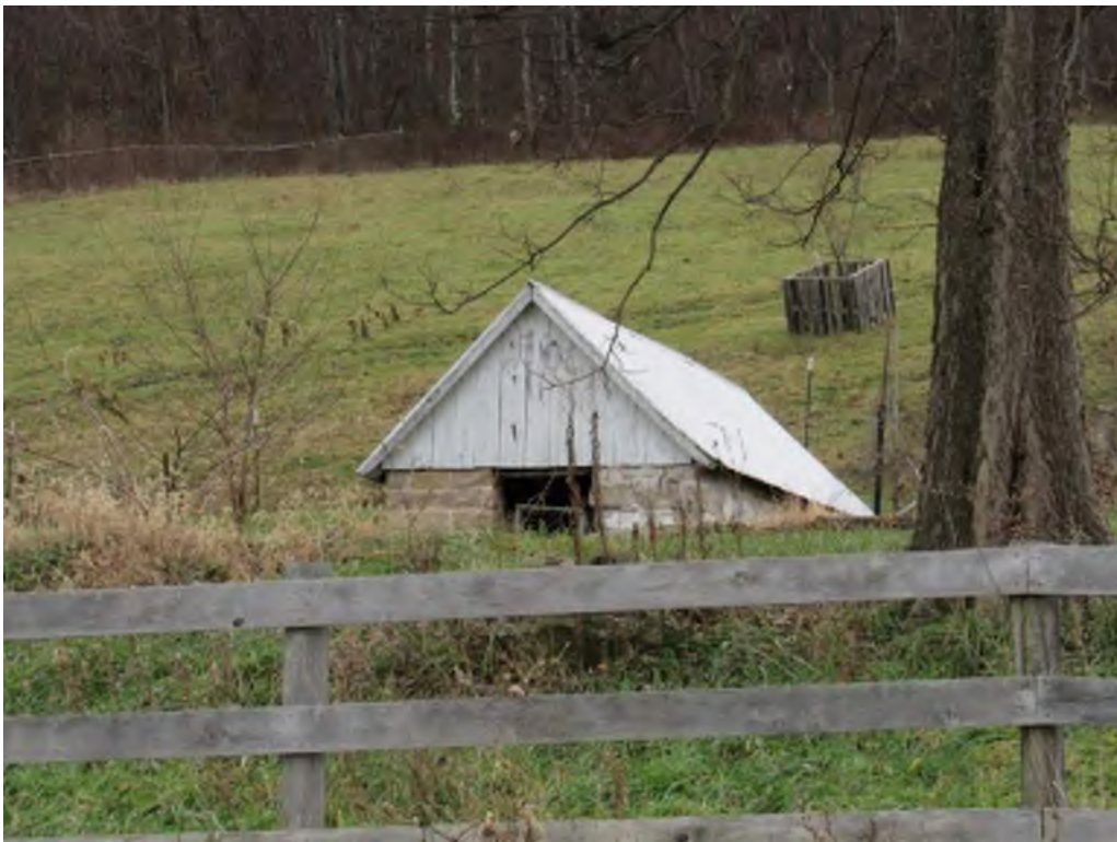
Photograph 2. Root cellar, facing east (Markosky 2018-12-04)
