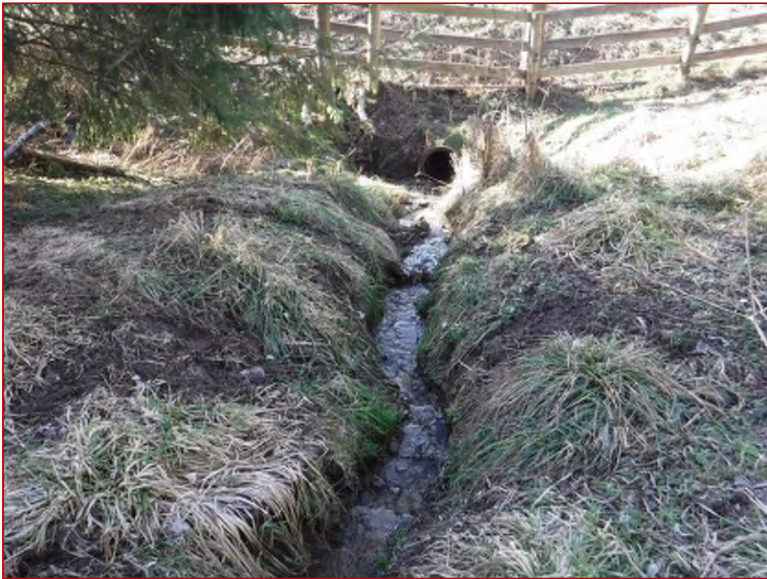
Photo 32: STR 9 - Facing Downstream (2.4.19)
