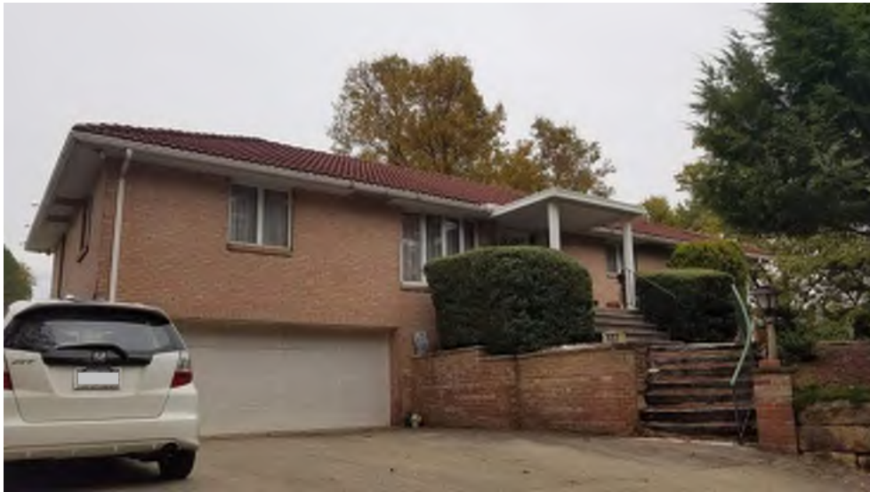
Photograph 1. MG-2642 / Ranch at 851 Greenbag Road, west and south (front) elevations, facing northeast
