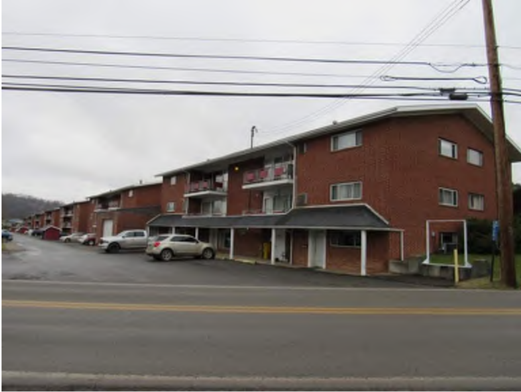
Photograph 31. MG-2655 / Mountain View Manor, Morgantown, Monongalia County Overview of buildings, facing west
