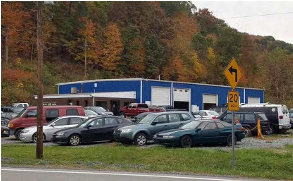
Photograph 1. North (front) and west elevations, facing southeast
