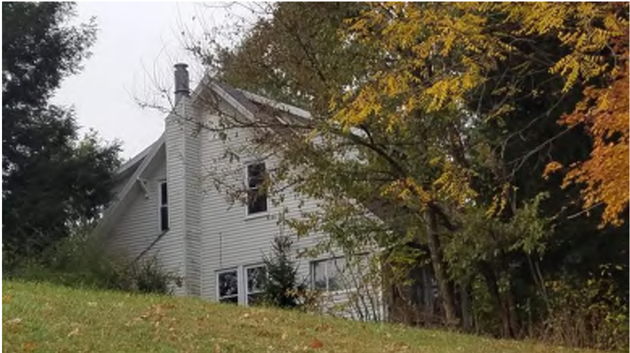
Photograph 2. East and north (front) elevations, facing southwest
