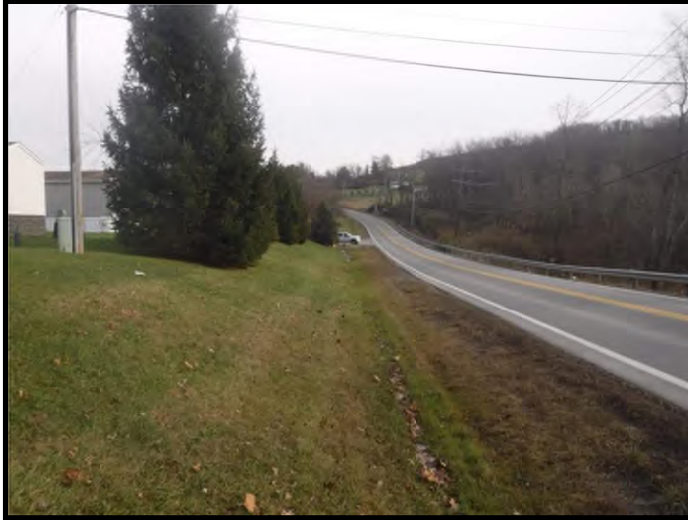
Photograph 29. View of cut slope in the study area, facing east.
