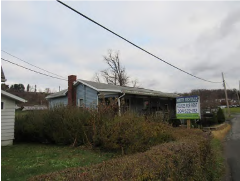
Photograph 1. Façade and southwest elevation, facing northeast (Markosky 2018-12-05)
