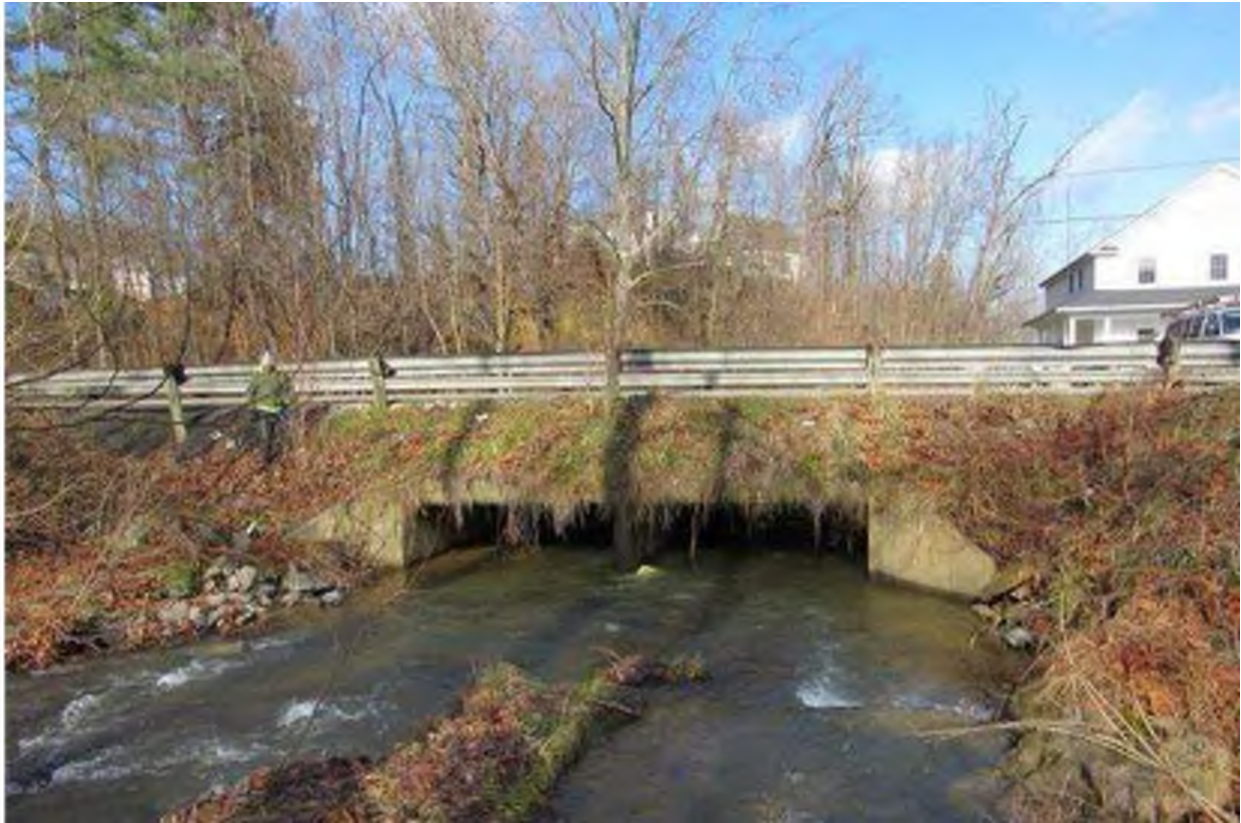
Photograph 3. South elevation of culvert, facing northeast (WVDOH 2018)
