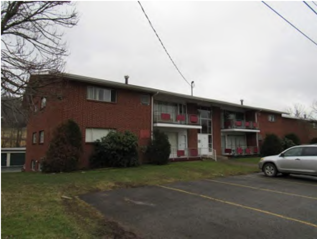
Photograph 1. Representative building, northwest elevation, facing southwest (Markosky 2019-02-05)
