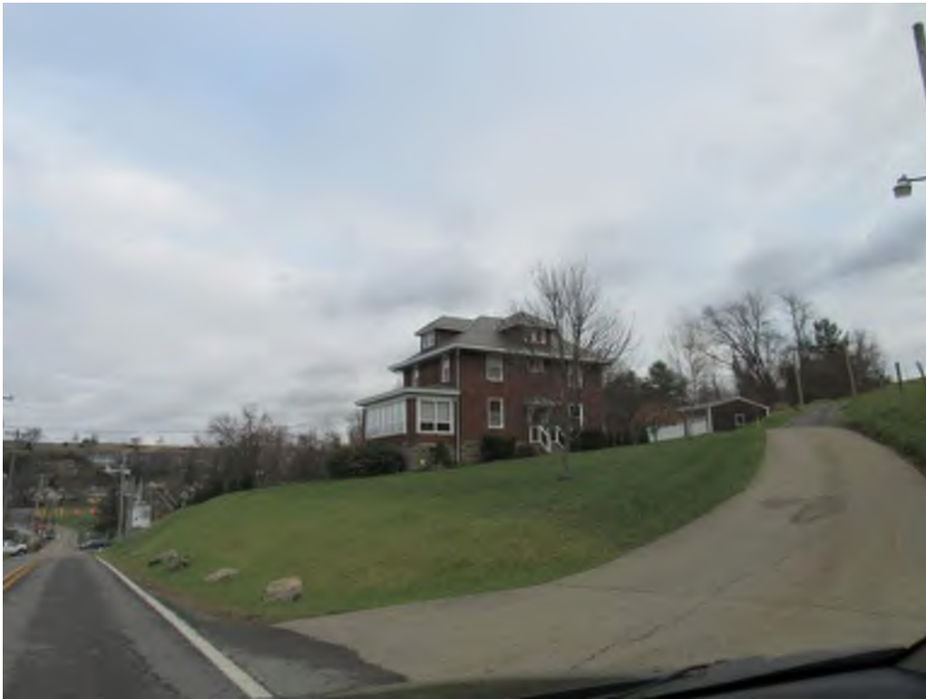
Photograph 1. Overview showing house and non-historic garage, facing northeast (Markosky 2018-12-04)
