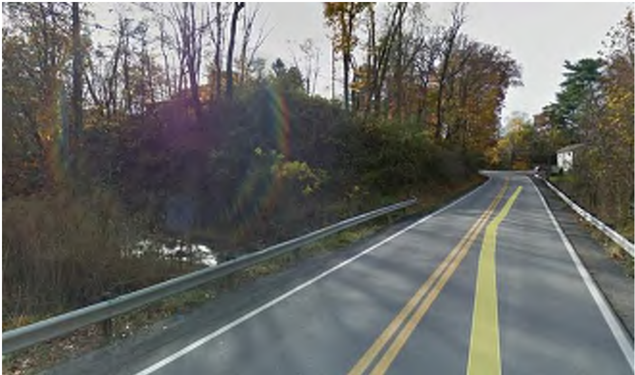
Photograph 1. Through view of culvert, facing southwest (Google Earth 2019)
