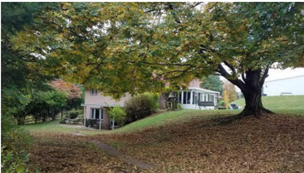
Photograph 2. MG-2642 / Ranch at 851 Greenbag Road, east and north (rear) elevations, facing southwest
