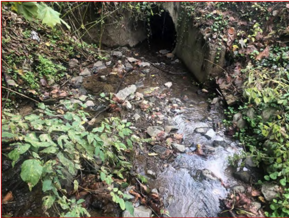
Photo 38: STR 10 (DS Point) - Facing Downstream (10.8.19)
