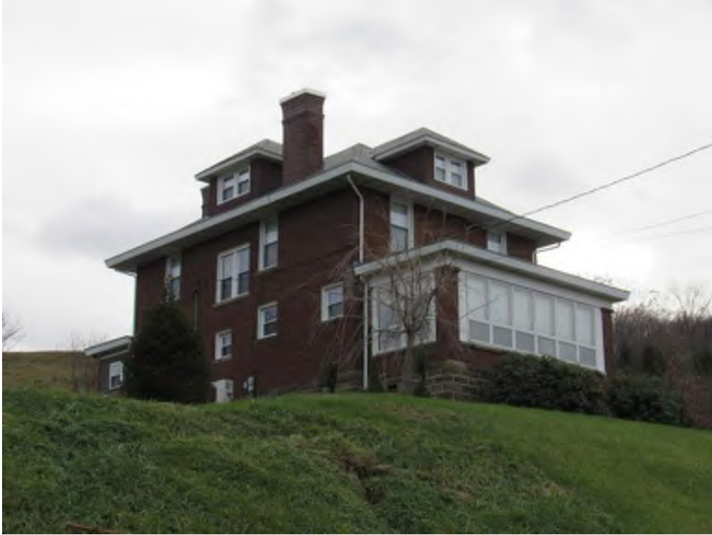
Photograph 21. MG-2647 / Anderson House, Morgantown, Monongalia County House showing enclosed front porch, facing southeast
