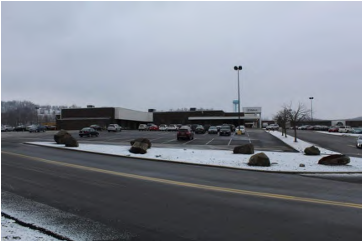
Photograph 6. MG-2643 / Mountaineer Mall, Morgantown, Monongalia County Overview, facing southwest
