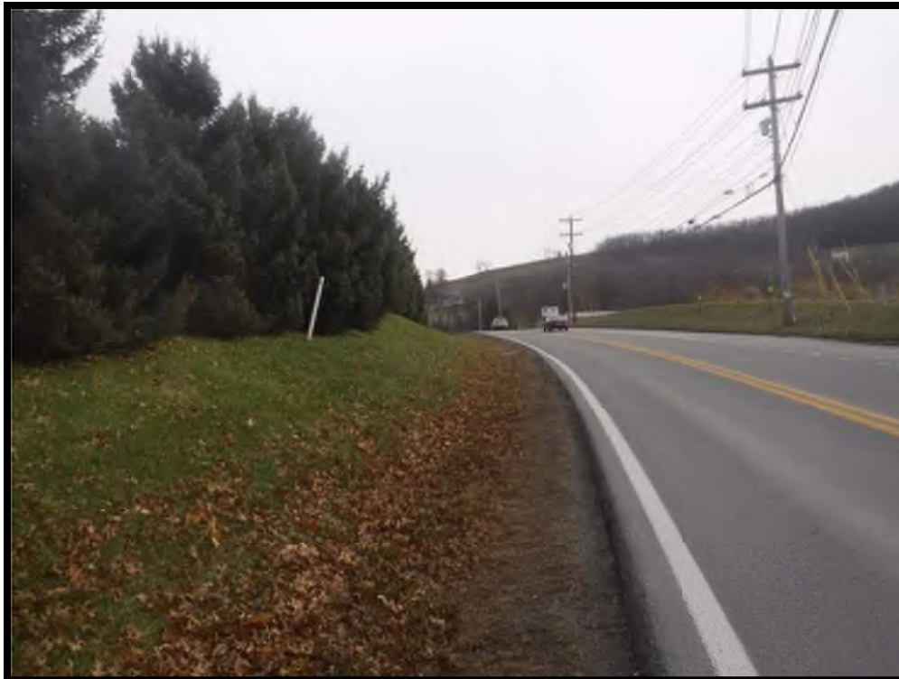
Photograph 28. View of cut slope in the study area, facing east.
