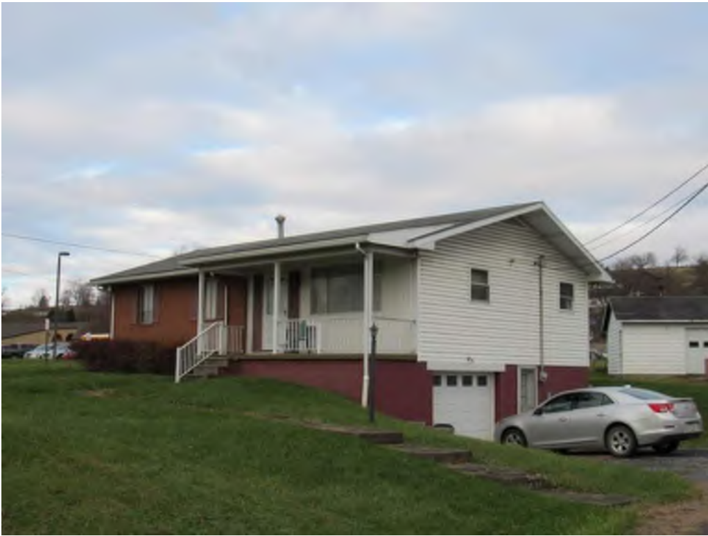
Photograph 1. House with integral garage, facing northwest (Markosky 2018-12-04)
