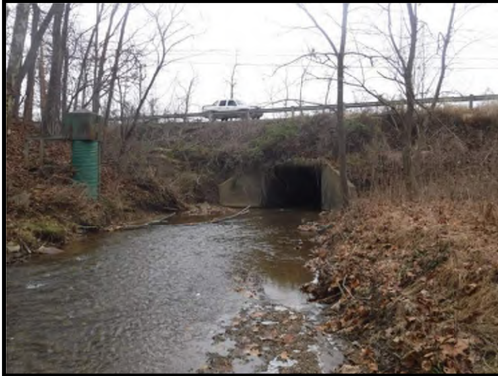
Photograph 19. General view of the study area, facing north.
