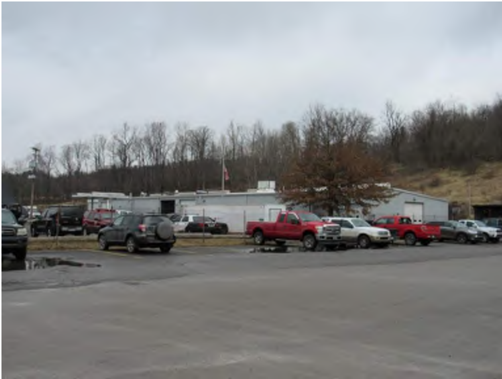
Photograph 1. Southwest and southeast elevations, facing north (Markosky 2019-02-05)
