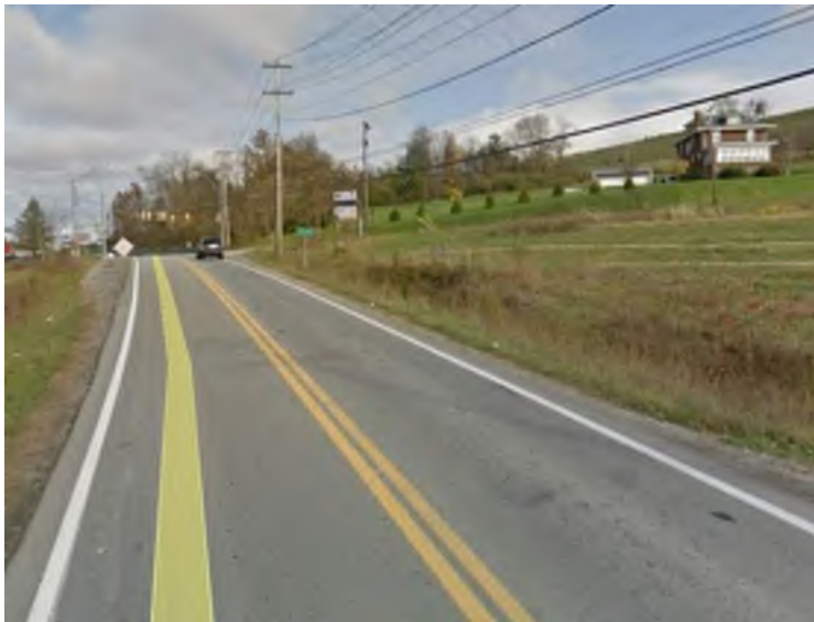
Inset 6. Overview of Project APE showing MG-2647 / Anderson House with farmland (right) and intersection of Greenbag Road and Dorsey Avenue / Kingwood Pike (left), facing northeast (Google Earth 2018)
