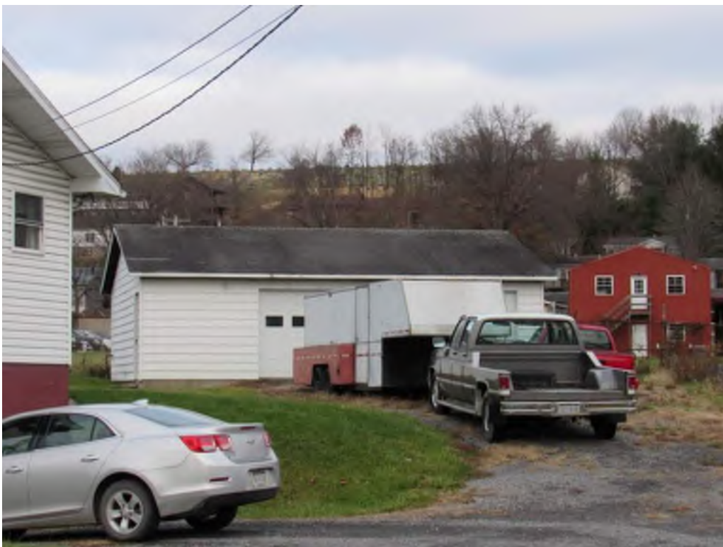
Photograph 2. Garage north of house, facing northwest (Markosky 2018-12-04)
