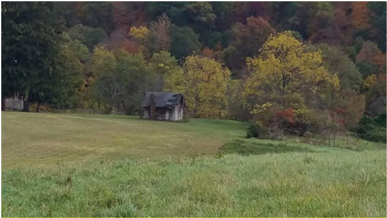
Photograph 5. West (side) elevation of ca. 1940 outbuilding, facing east.
