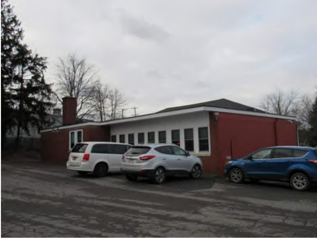
Photograph 27. MG-2651 / Dorsey School, Morgantown, Monongalia County Rear addition, facing southwest
