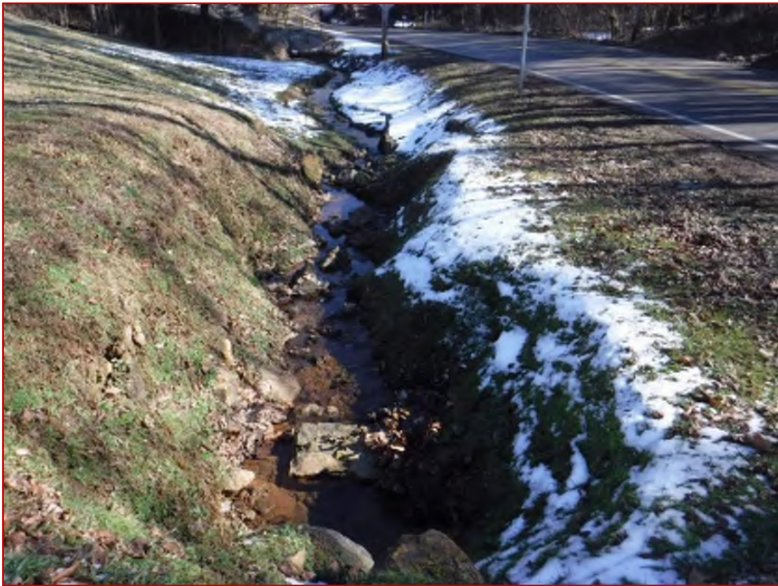
Photo 36: STR 11- Facing Downstream (2.4.19)
