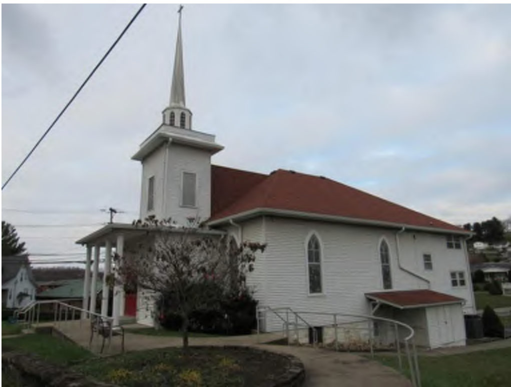
Photograph 2. Northeast elevation, facing northwest (2018-12-04)
