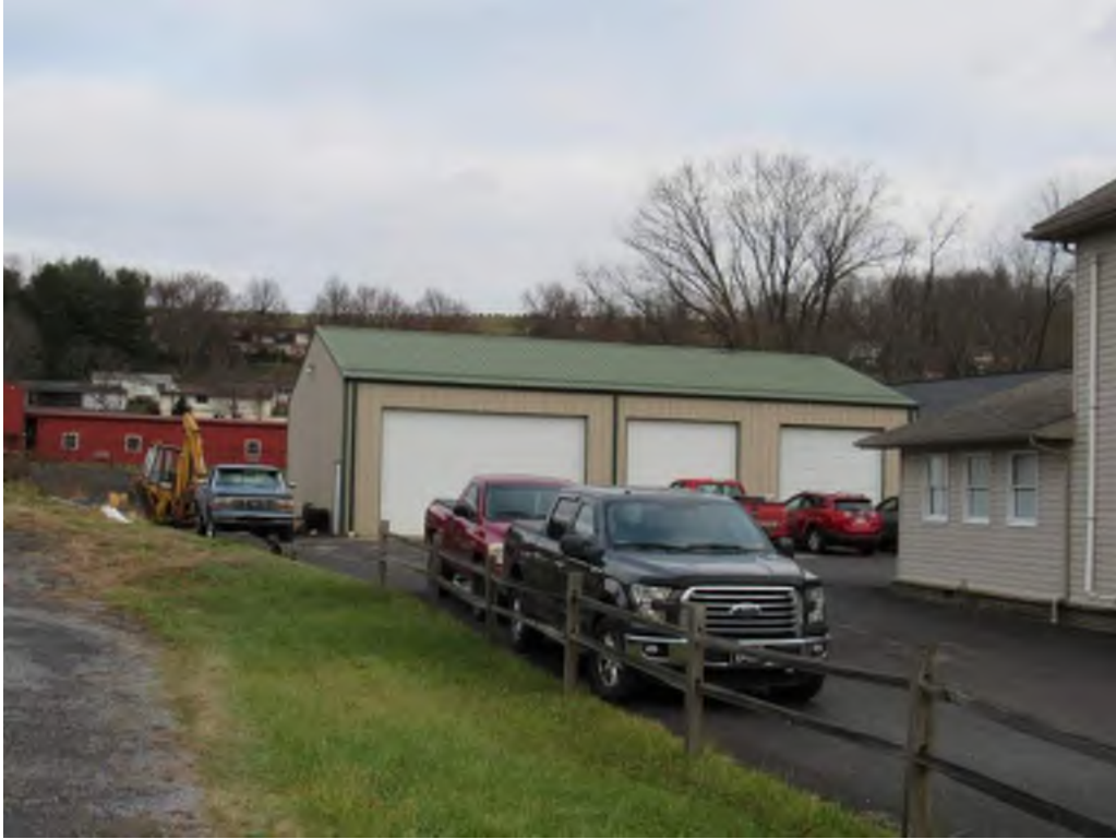
Photograph 37. MG-2659 / House at 703 Greenbag Road, Morgantown, Monongalia County Garage north of house, facing north
