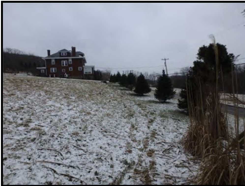
Photograph 83. View of Test Area 10, facing south.
