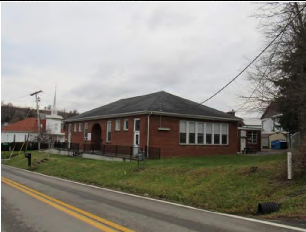
Photograph 1. Façade and south elevation, facing northeast (2018-12-05)
