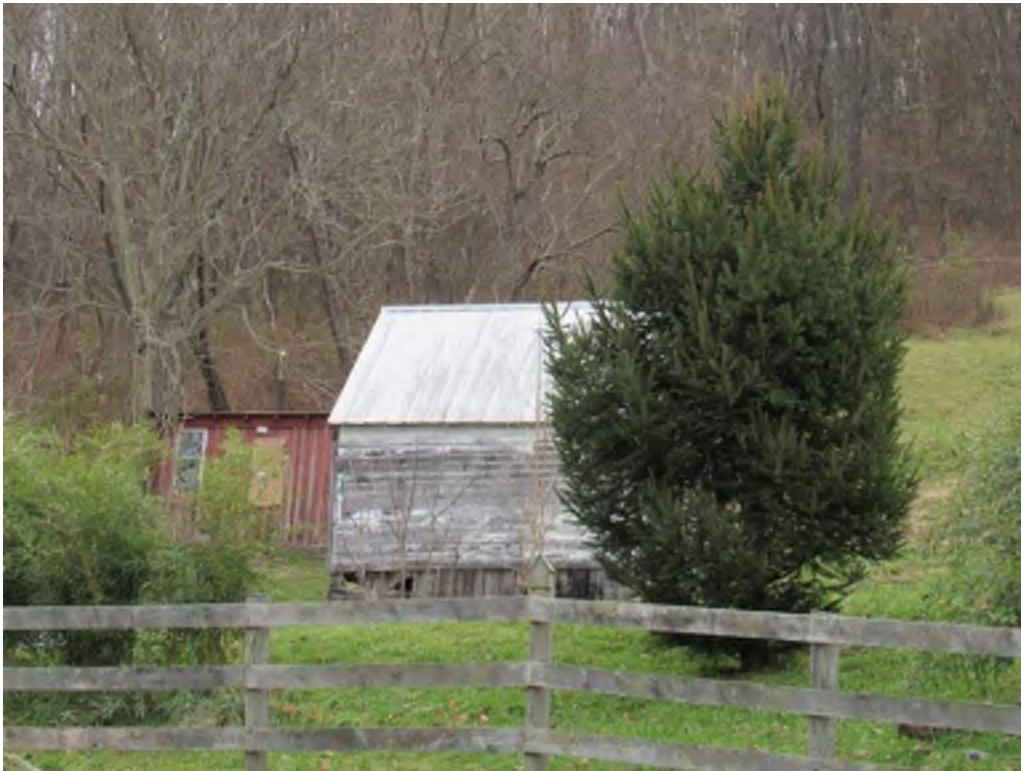
Photograph 3. Shed #1 (foreground) and Shed #2 (background), facing east (Markosky 2018-12-04)
