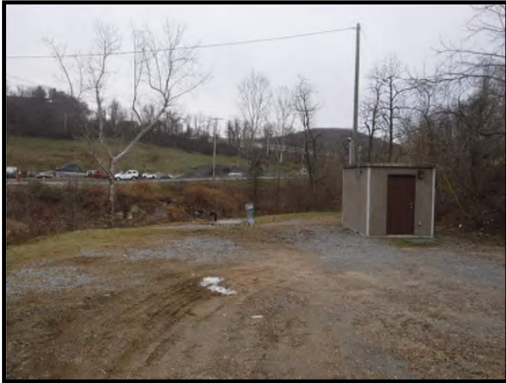
Photograph 11. General view of the study area, facing east.
