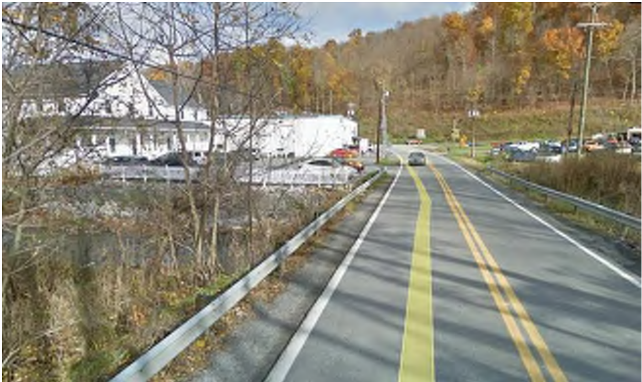
Photograph 2. Through view of culvert, facing northeast (Google Earth 2019)
