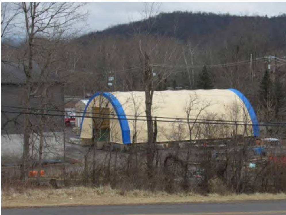
Photograph 2. Prefabricated outbuilding, facing southeast (Markosky 2019-02-05)
