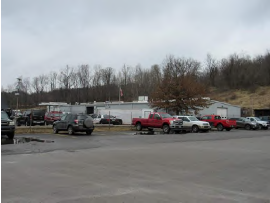
Photograph 9. MG-2644 / Morgantown City Garage, Morgantown, Monongalia County Southwest and southeast elevations, facing north
