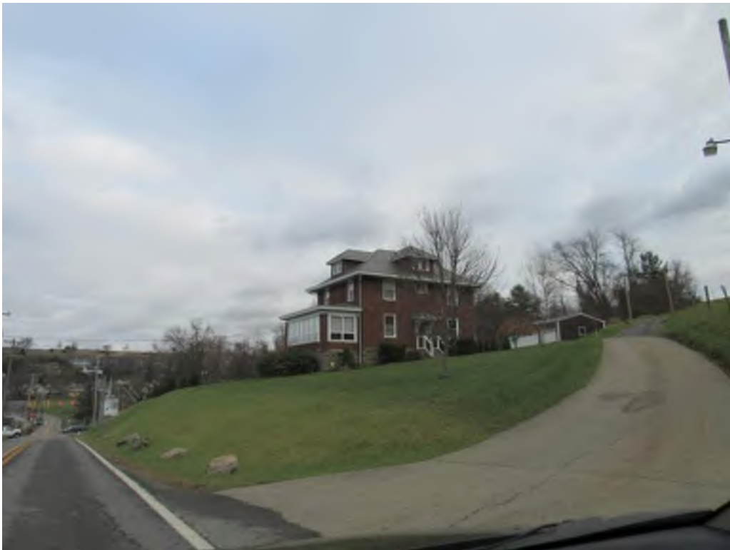
Photograph 20. MG-2647 / Anderson House, Morgantown, Monongalia County Overview showing house and non-historic garage, facing northeast
