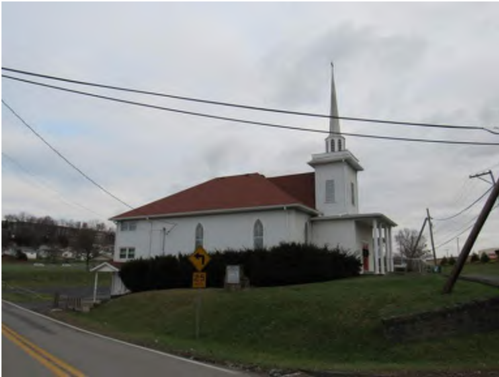
Photograph 1. Façade and rear addition (left), facing northeast (2018-12-04)
