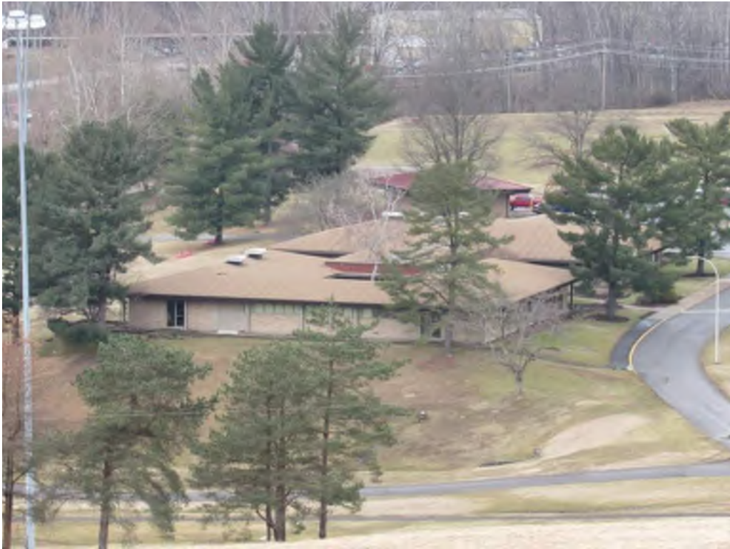
Photograph 14. MG-2645 / FCI Morgantown Kennedy Center/R.F.K. Youth Center, Morgantown, Monongalia County Representative building, facing west
