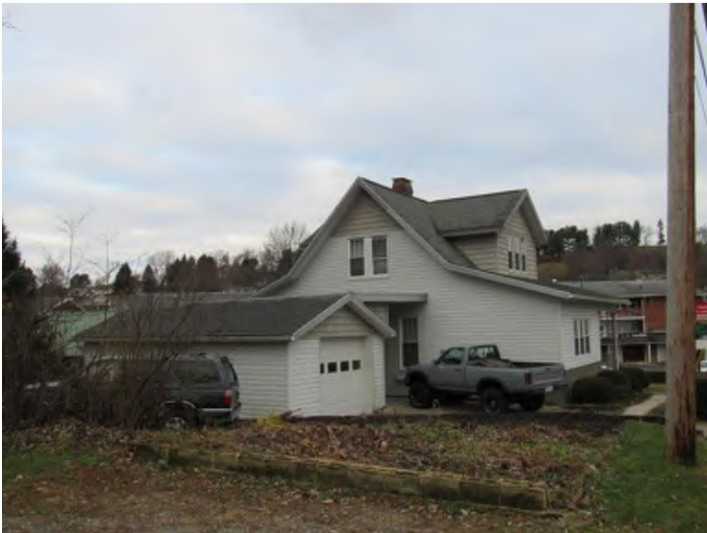
Photograph 28. MG-2652 / House at 1432 Dorsey Avenue, Morgantown, Monongalia County House and garage, facing northwest
