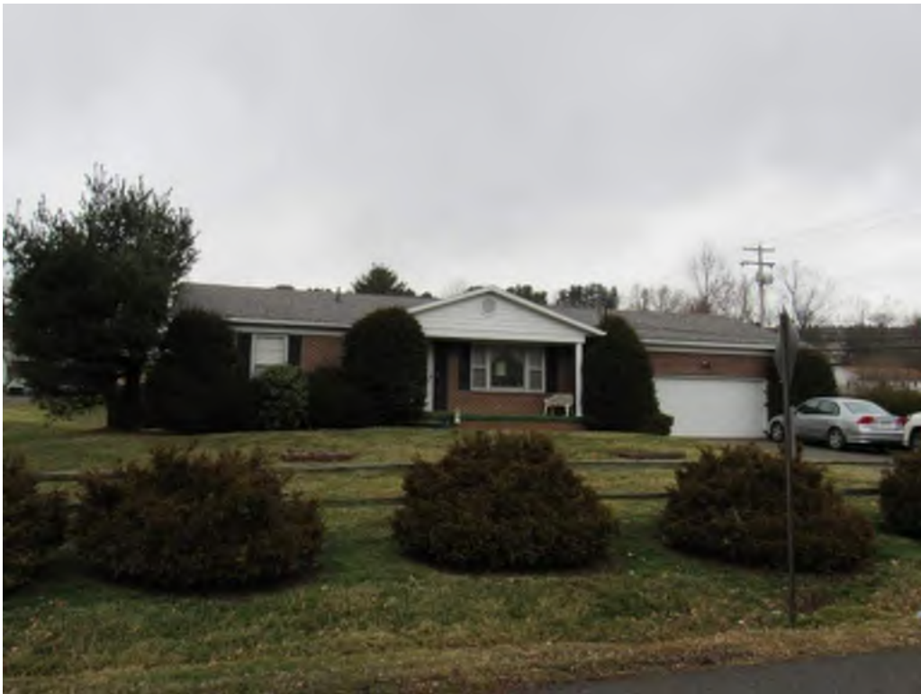
Photograph 32. MG-2656 / House at 500 Parkway Drive, Morgantown, Monongalia County House and garage, facing north
