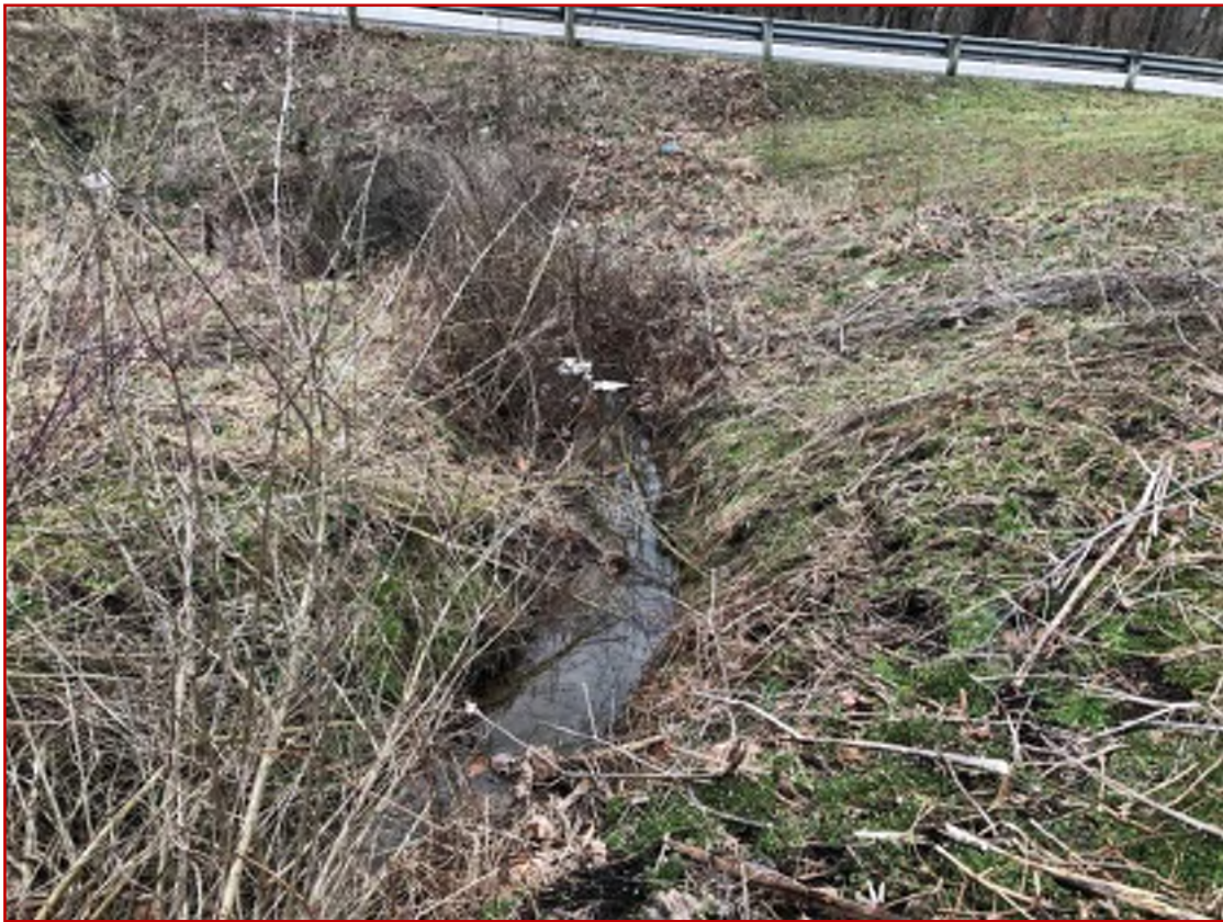
Photo 26: STR 6 - Facing Downstream (3.13.19)
