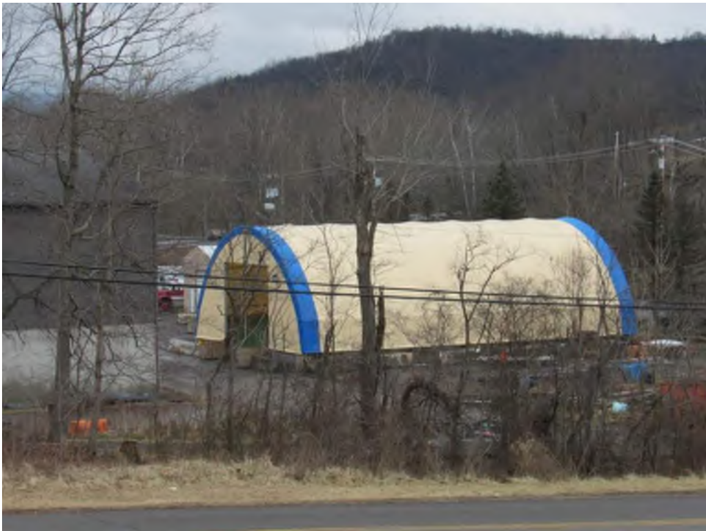
Photograph 10. MG-2644 / Morgantown City Garage, Morgantown, Monongalia County Prefabricated outbuilding, facing southeast
