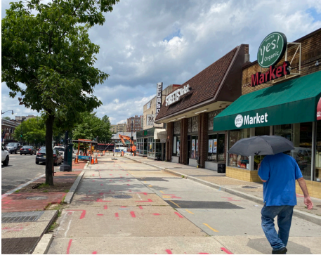
7 Temporary pedestrian-only path outside of storefronts
