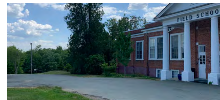
(above) An existing field on the site, looking toward the stream, and the Old Crozet School building.
