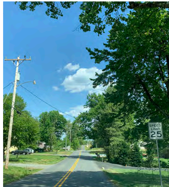
(Above) A section of Park Road, which currently lacks sidewalks. Park Road was identified by community members as a top priority for future sidewalks projects.
