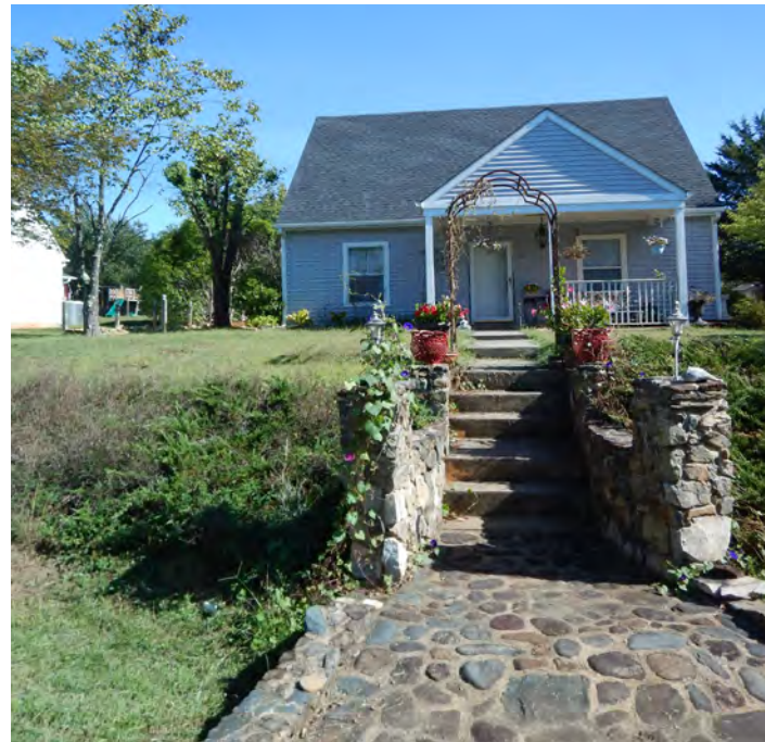
(Above) An example of a small, single-family cottage in Crozet.
