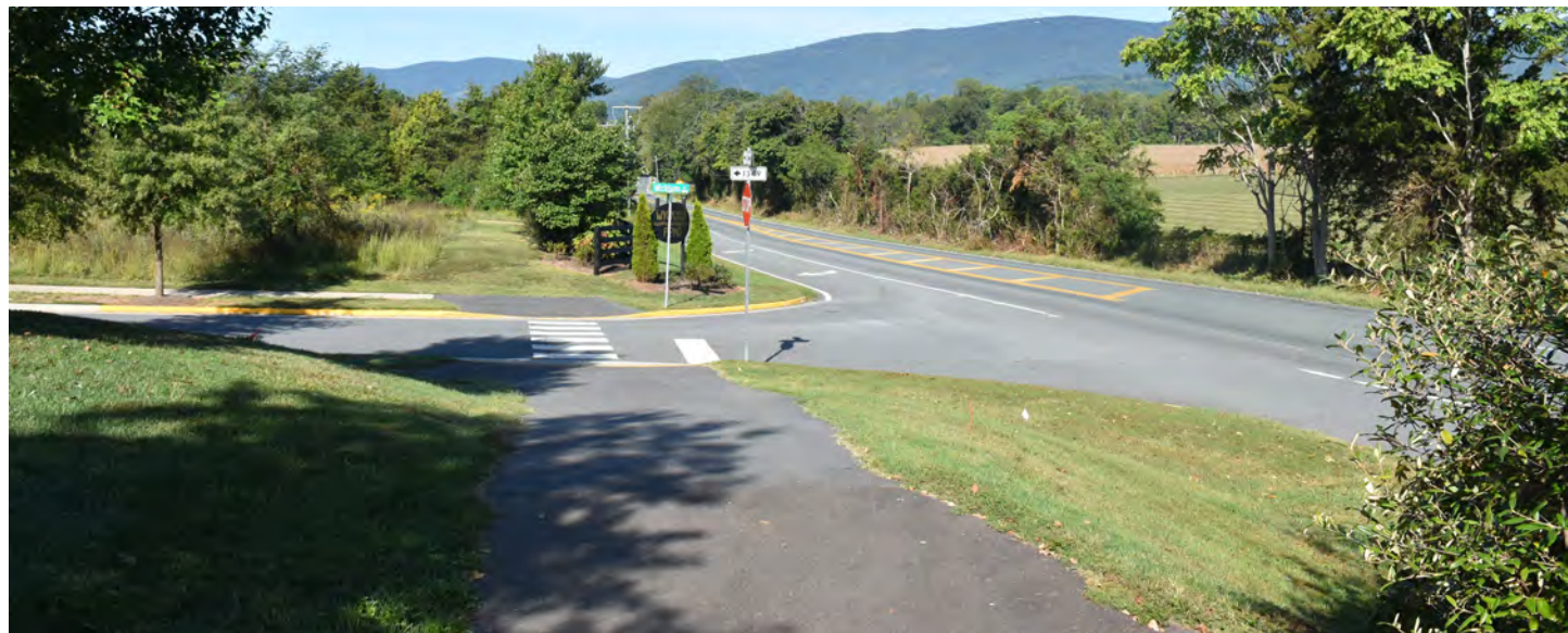
Above: The existing portion of the Three Notch'D Road Shared-Use Path, which is along the front of Wickham Pond.
