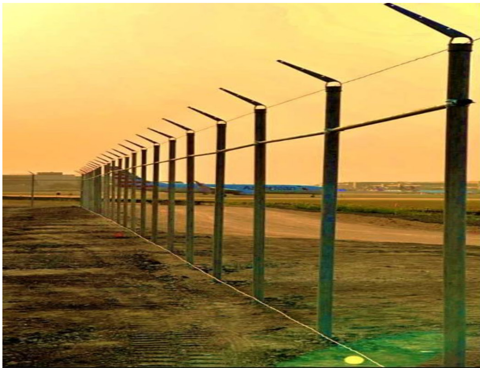
Installation of AOA Security Fence
