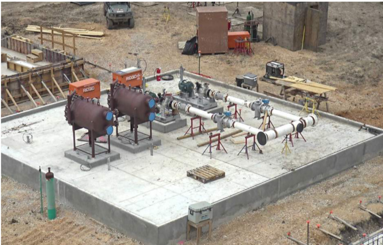
Piping and equipment installation
