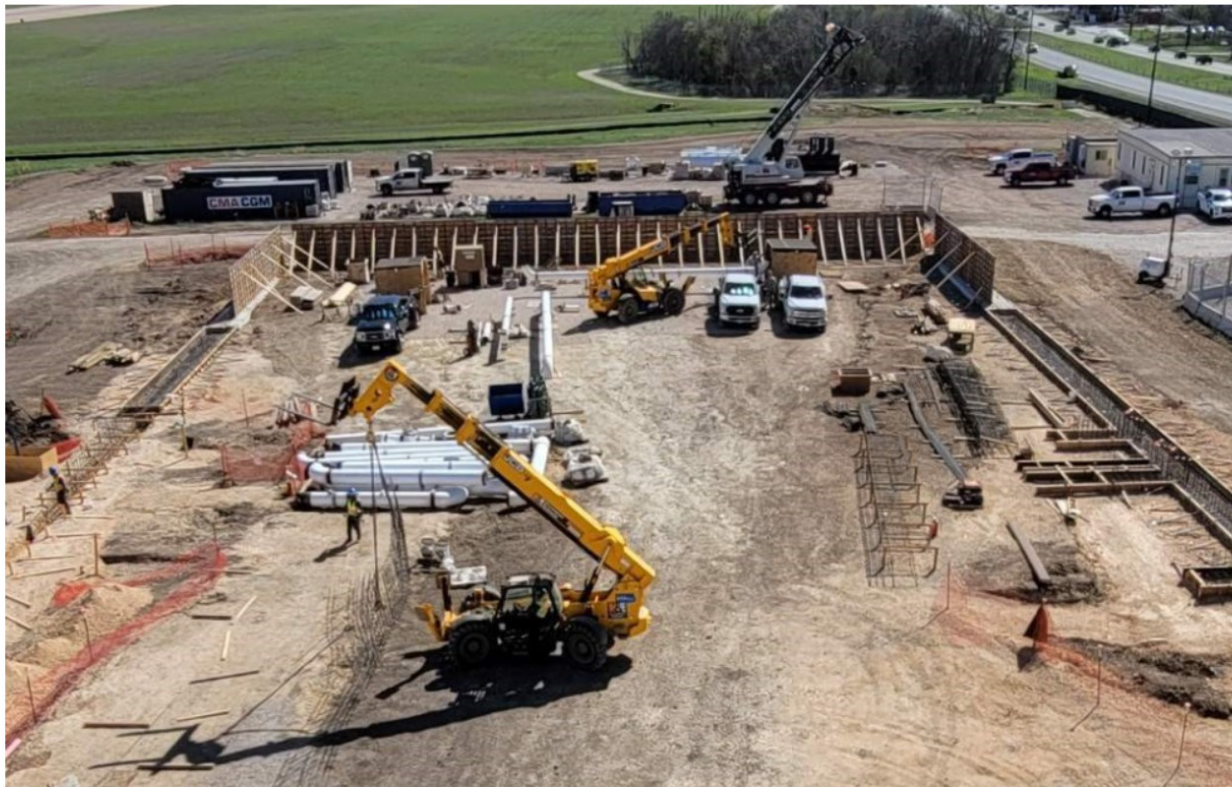
Preparing to pour concrete for the tank containment walls
