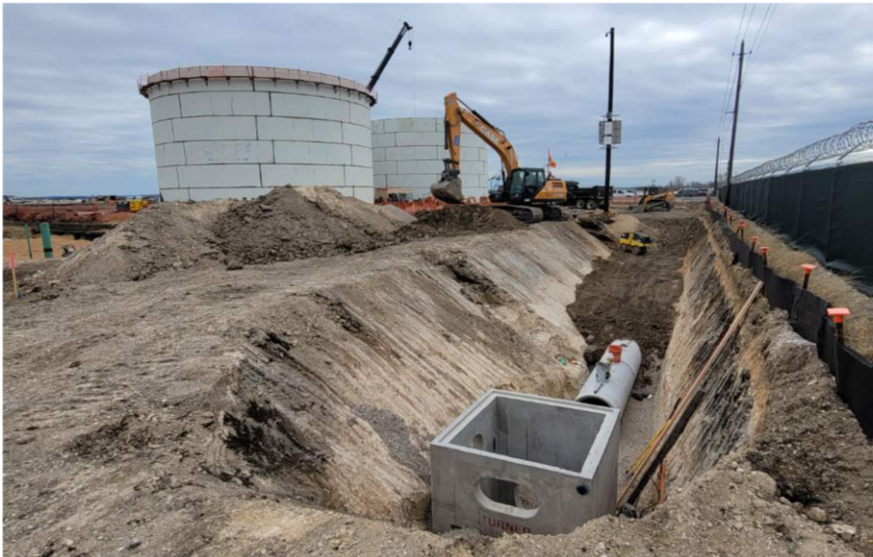
Installation of stormwater line in progress
