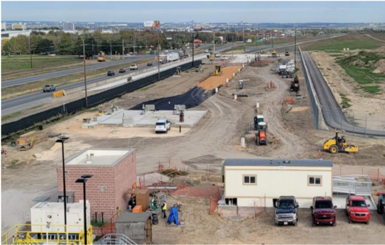
Site progress - North view
