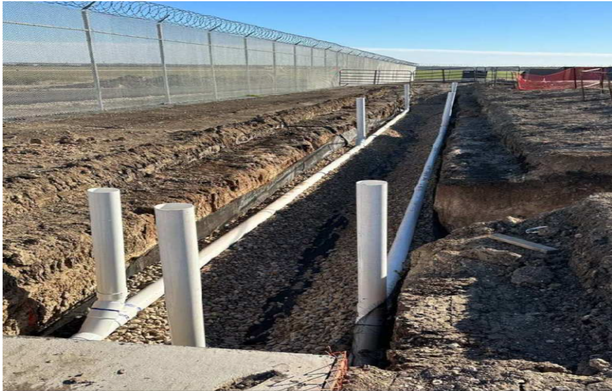
Rain Garden Construction
