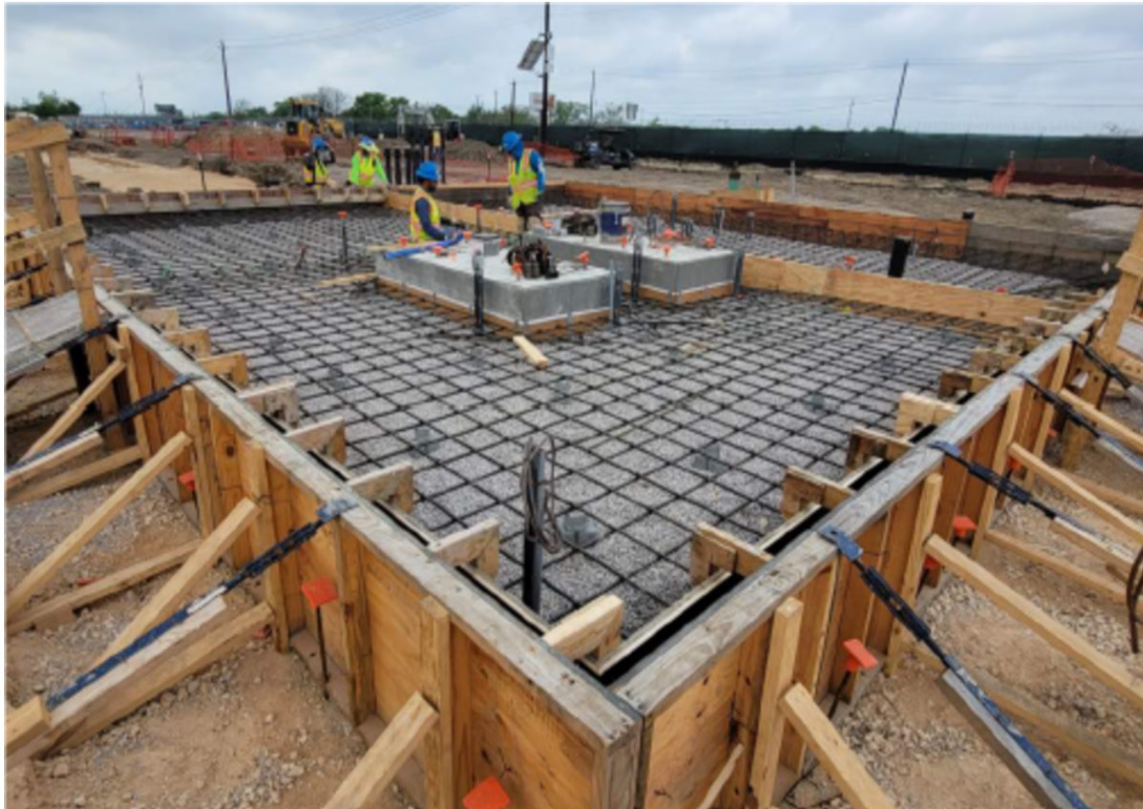
Tank containment walls under construction
