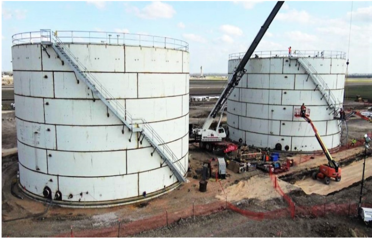
Tank steel wall installation
