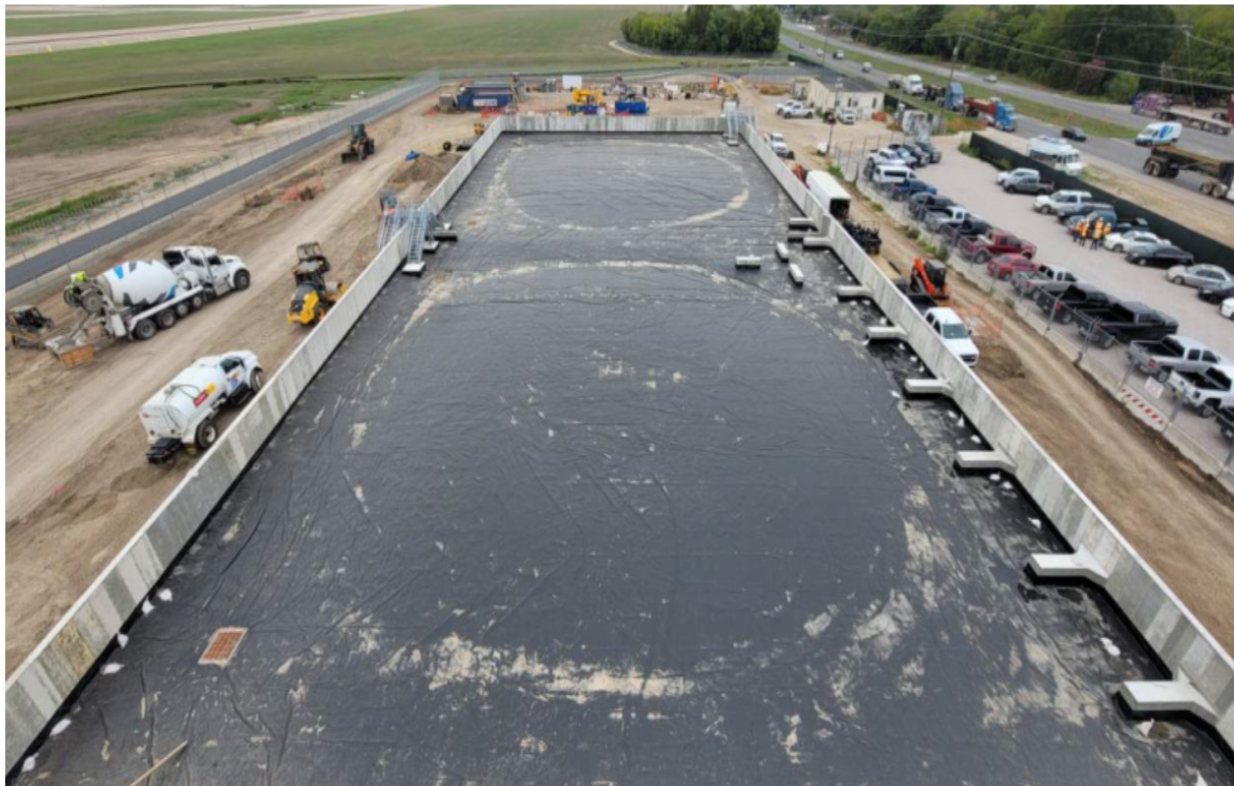
Site progress - North view
