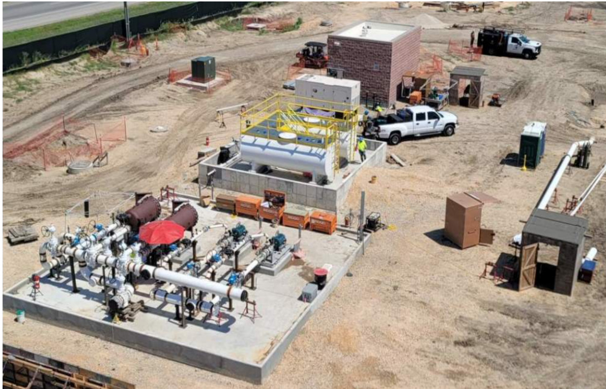
Installation of fueling equipment
