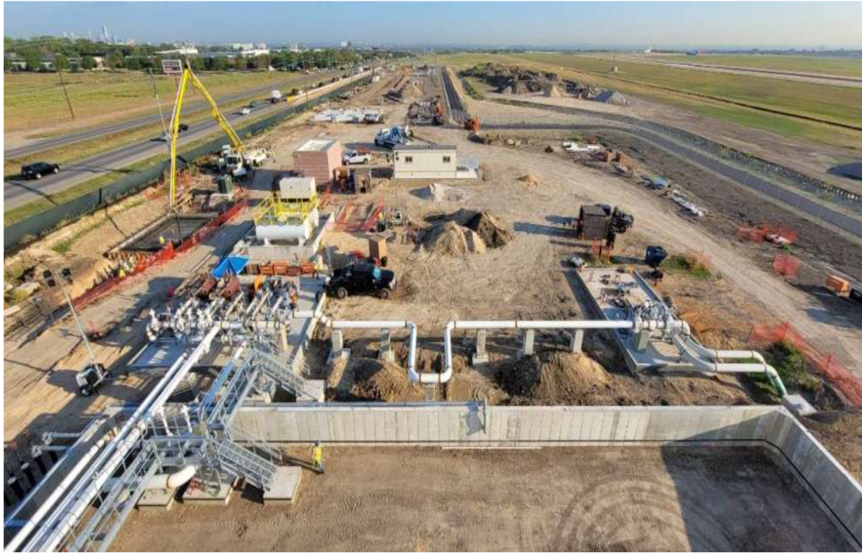
Site progress - North view
