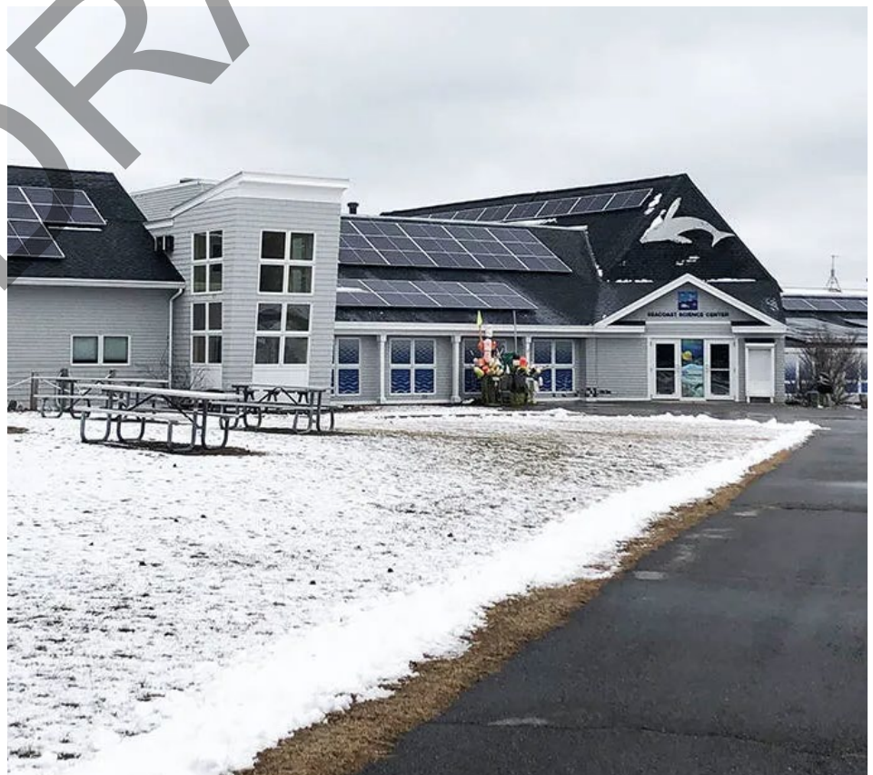
Above: Solar panels on the roof of the Seacoast Science Center in Rye, NH
